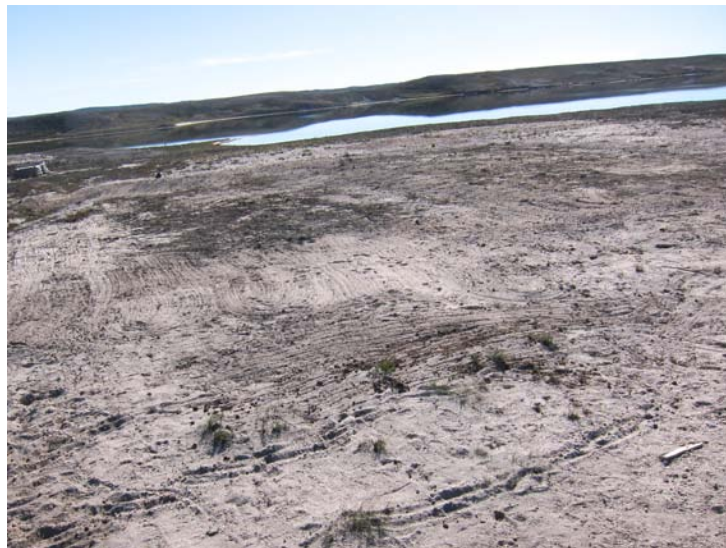
Figure 11. Demonstrating leveling and contouring to original state at the site of the fuel berms. July 2013.
