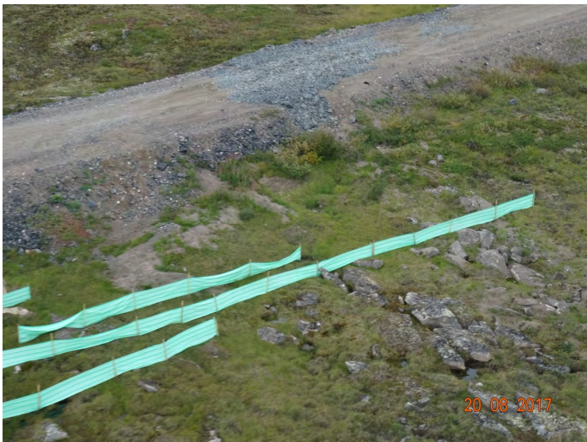
Road Repairs and Silt Fencing (August 2017)
