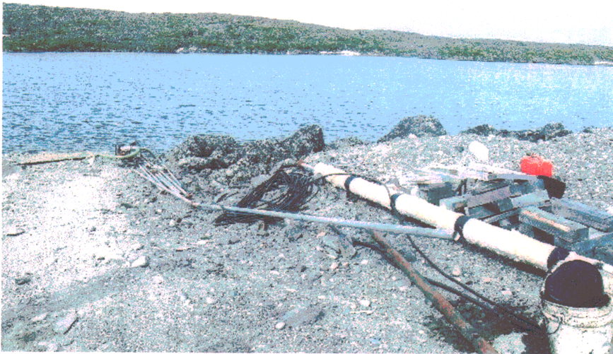
Figure 1. The freshwater intake at West Lake that was under repair at the time of the Inspection.
