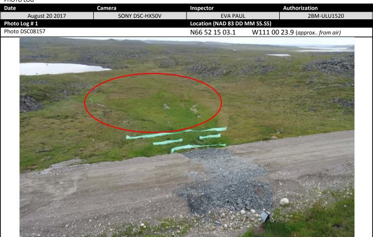
Description: Aerial view of one large wash-out area that has been backfilled (presumably with ore based on Ms. Lewis' information. Silt fences may mitigate further sediment from the road, but none are present between the existing sediment trail and the pond.
