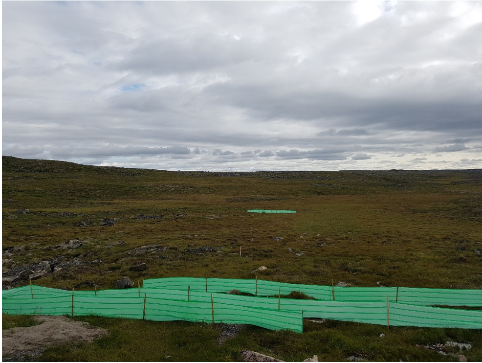
Photo 3: Additional silt fence installed further downstream at Culvert 6 as requested by the INAC inspector
