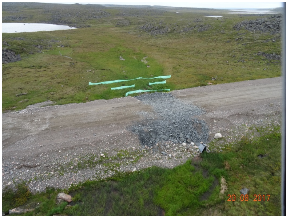
Photo 2: Silt Fences installed downstream of repaired road at the location shown in Culvert 7
