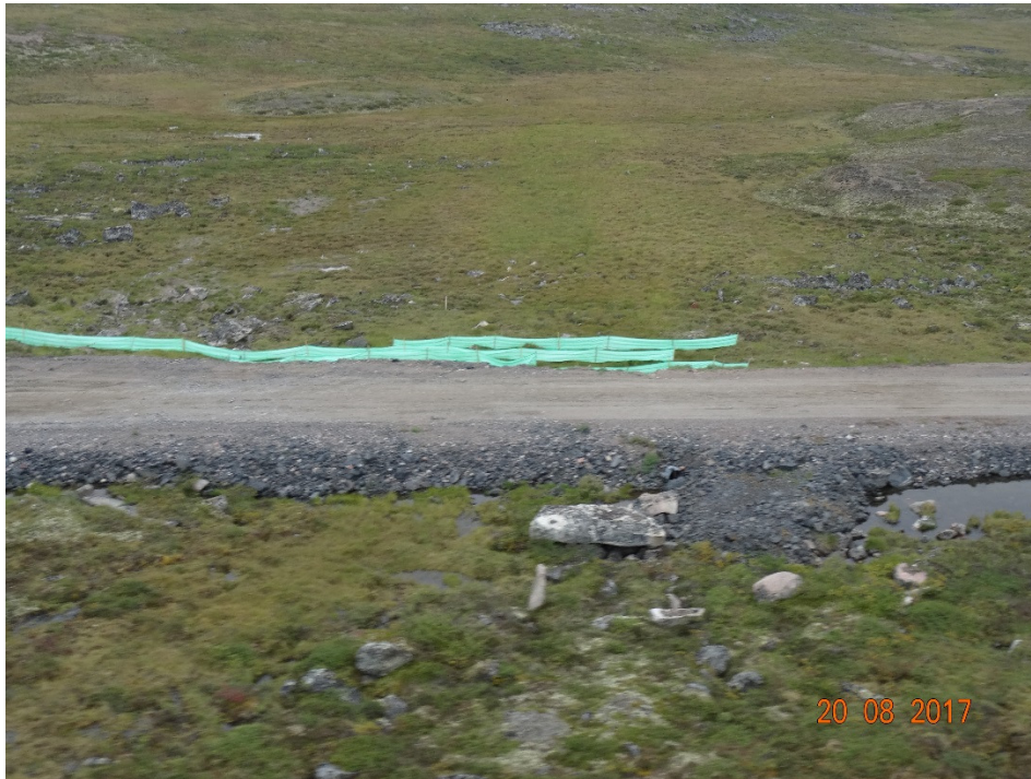
Photo 1: Silt Fences installed downstream of repaired road at the location shown in Culvert 6
