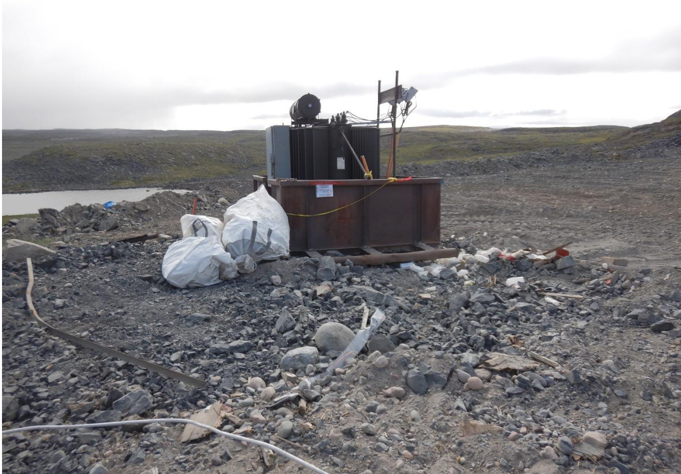
Description: Old PCB Transformer, contains NO Oil, to be cleaned in 2022 then placed into Land Fill
