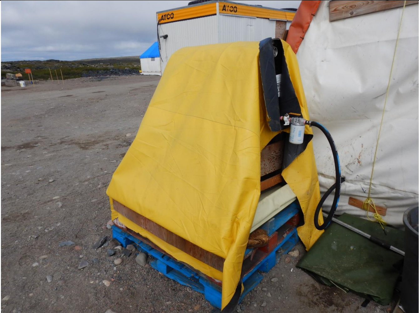
Description: Typical Secondary Containment of Fuel Drum outside most Tent Structures – Very Nice
