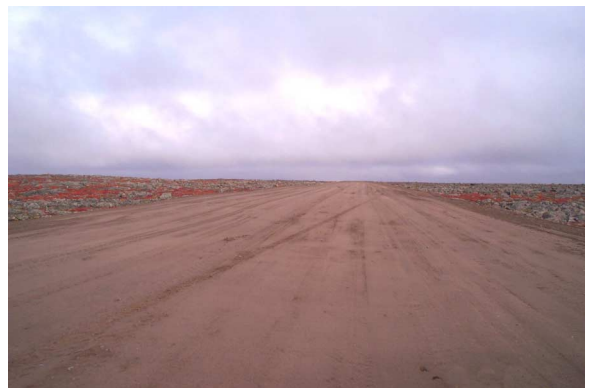
Photo 6 - Airstrip graded and packed
