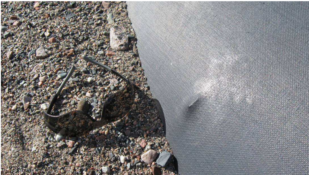
Typical Small Tear in Liner
