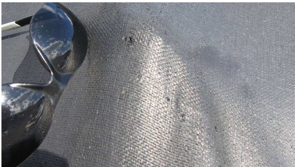
Typical Small Tear in Liner
