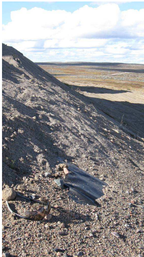
One Area of Exposed Liner on Downstream Slope
