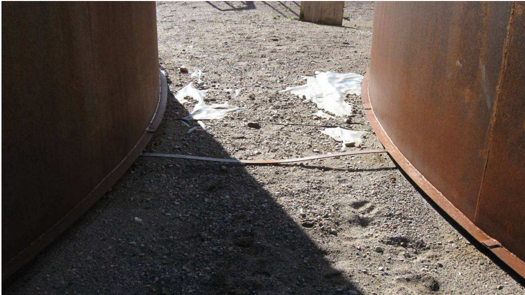
Exposed Liner Between Tanks
