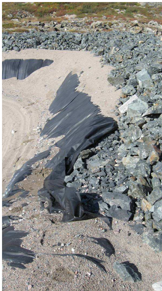
Exposed and Loose End of Liner
