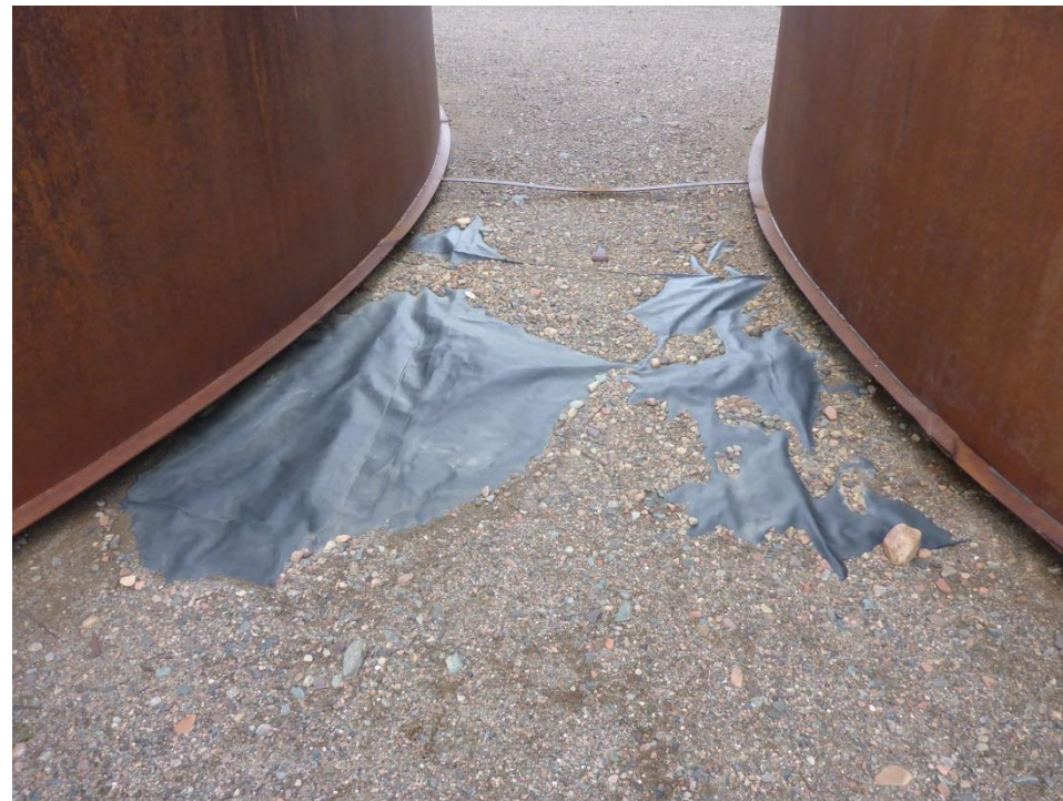
Photo 5: Close up view of the exposed liner between the 2 large tanks in Camp 3 fuel tank farm.
