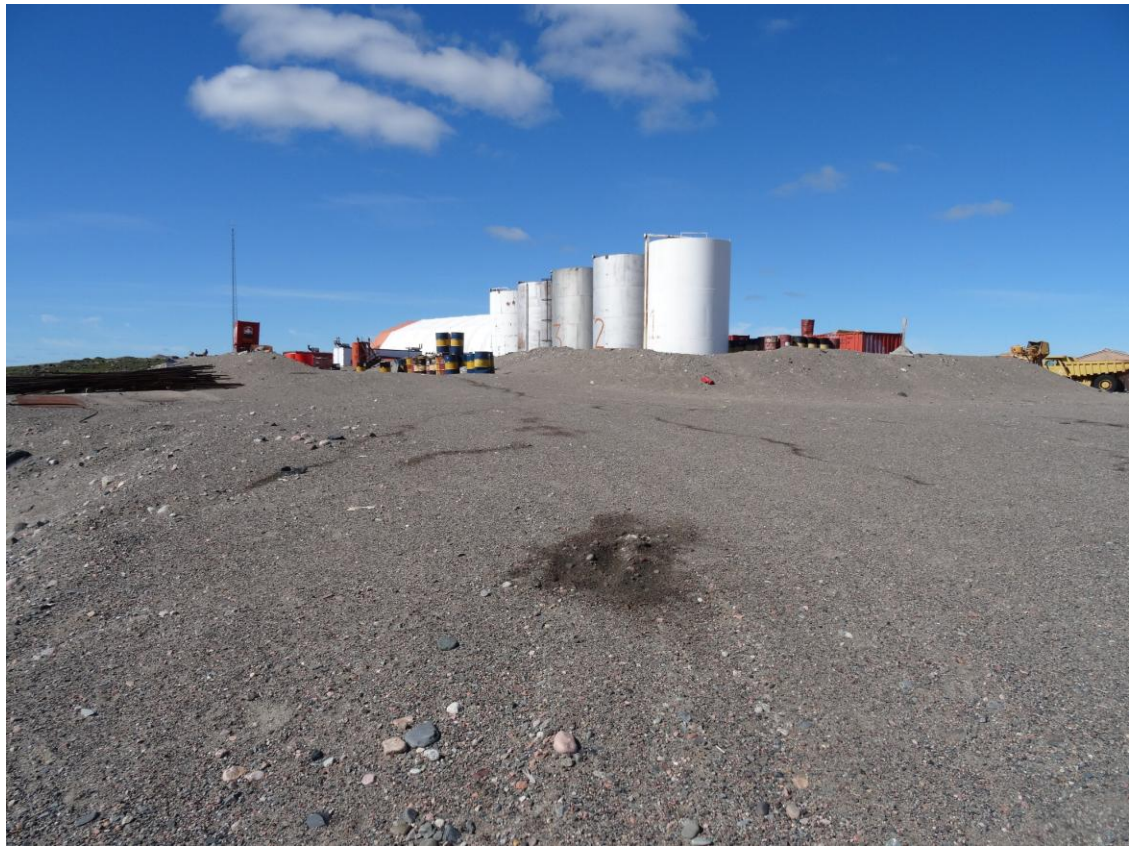
Figure 9. Fuel/barrel storage area to east of tank farm. Note staining running downhill from the lined area.
