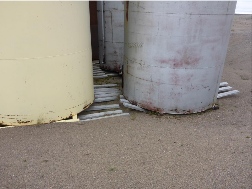
Photo 9: Close up view of the broken cribbing underneath the leaning tanks.
