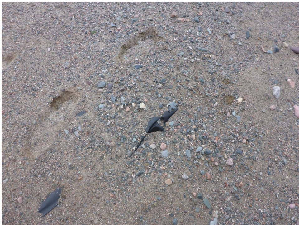
Photo 4: Close up view of the damaged liner in the southern bank of the Camp 3 fuel tank farm.
