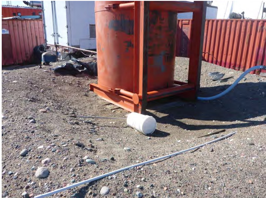
Photo 18: Looking west at the day use tank at Ulu. Note the exposed liner in the west bank.
