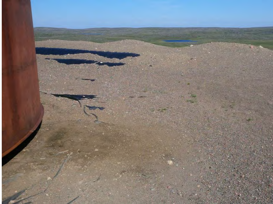
Photo 6: Looking at the exposed liner in the north bank of the Camp 3 fuel tank farm.
