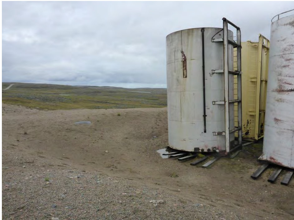
Photo 1: Looking north at one of the leaning tanks in the front of the Camp 3 fuel tank farm.
