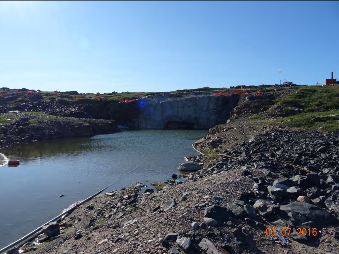
Description: Ulu portal, with piping and hoses visible, assumedly set up for a discharge.
