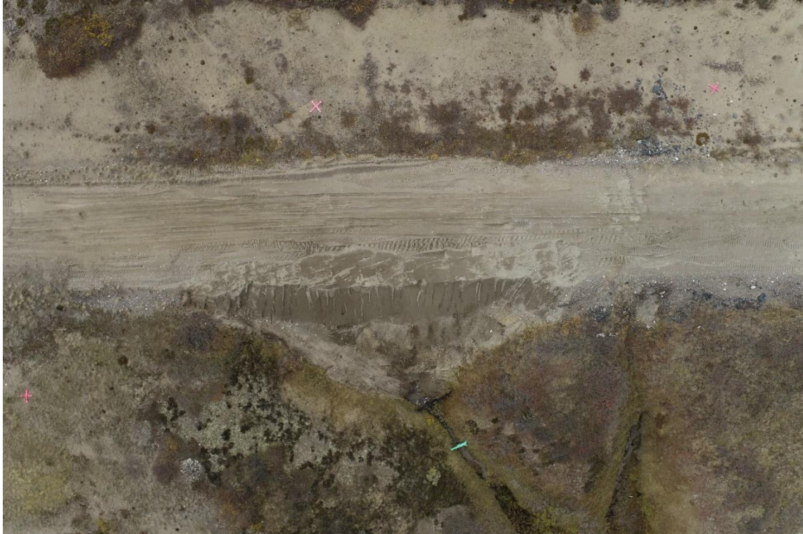
Photo 15. Completed road works near Camp 3
