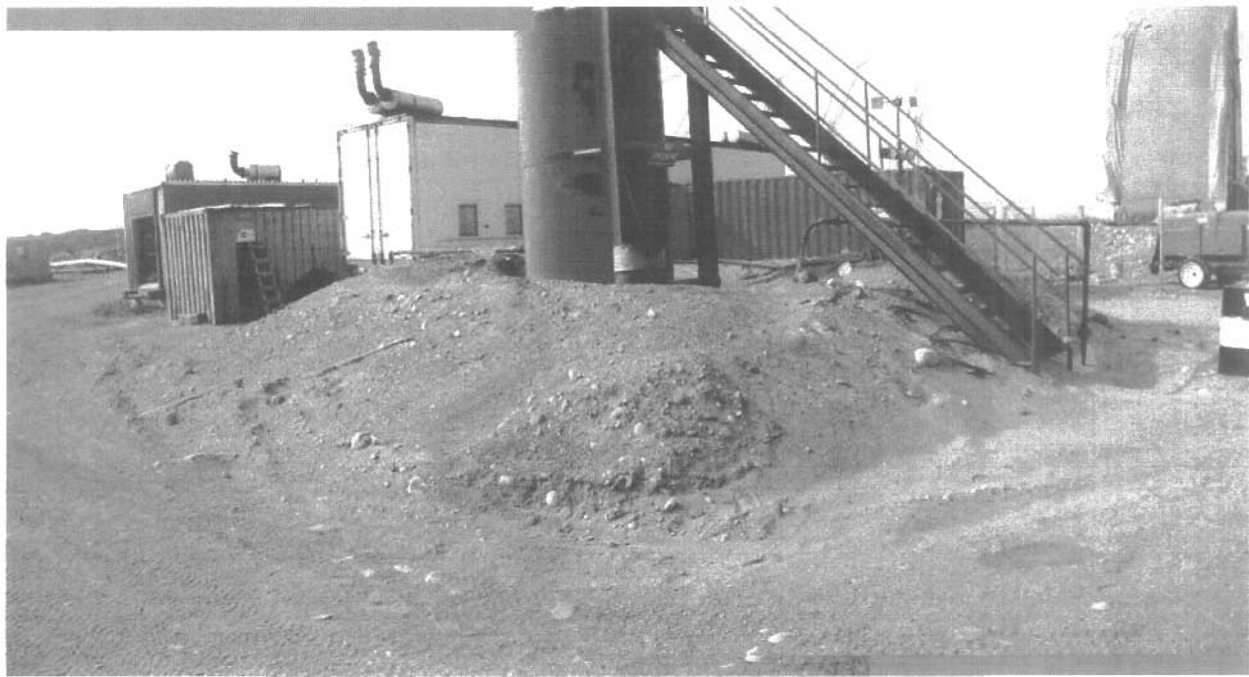
Photo shows the berm surrounding the day tank. It is a low berm approximately 1.2 m in height constructed of esker sand and gravel.
