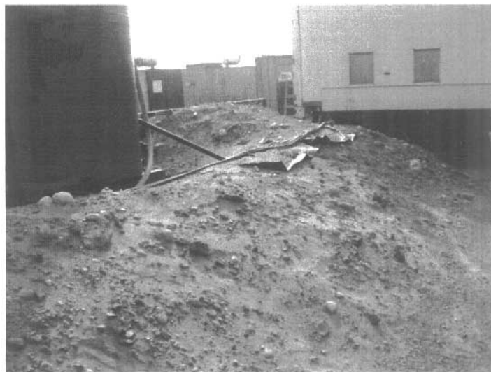
Photo shows the exposed edge of the liner.
