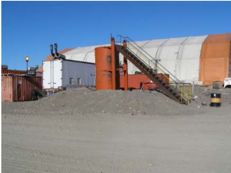
View of the small berm located around the Day Tank.
