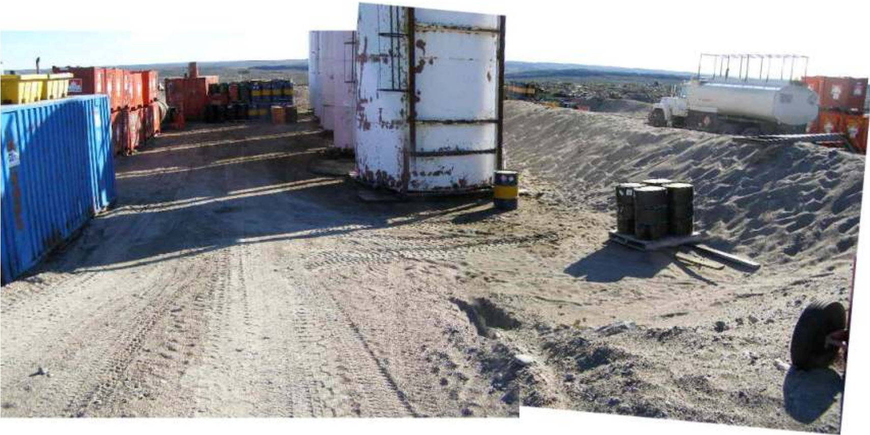
View of the inside of the containment berm, with no signs of erosion, exposed liner or standing water.
