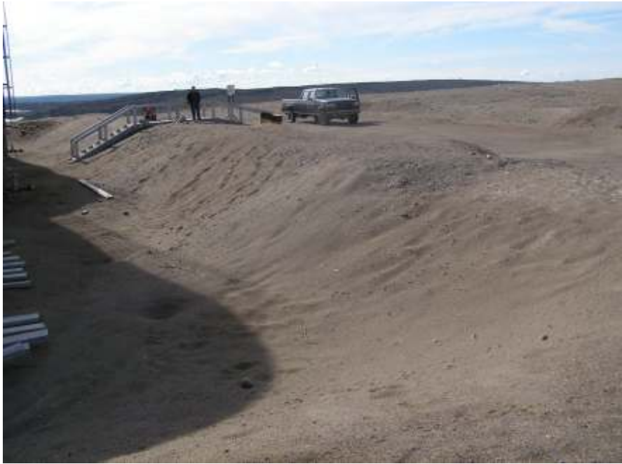
Shows the inside face of the west side berm. No signs of deformation, erosion, or exposed liner at this location.
