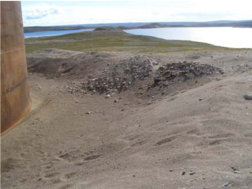
There are no signs of standing water inside the berm or any exposure of the liner at this area.
