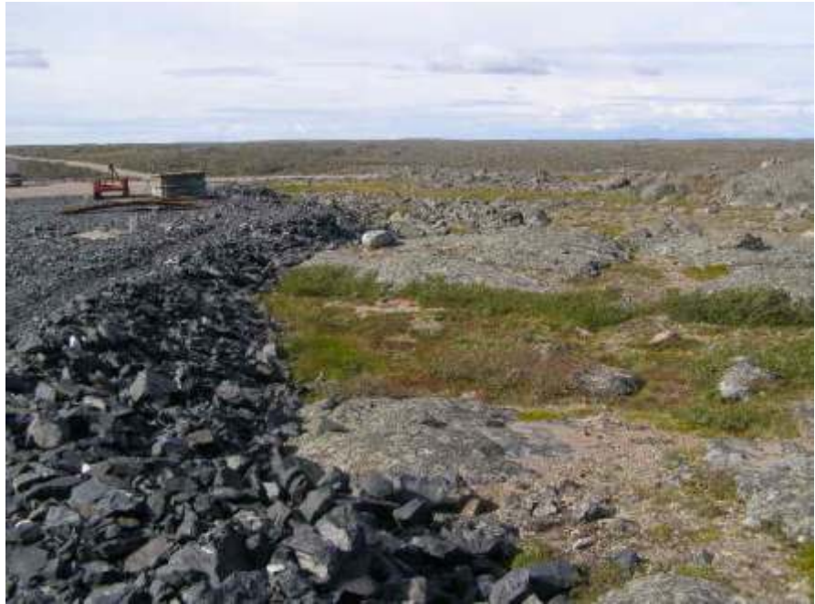
Shows a view along the northern edge of the pad; no signs of seepage or discharge were noted.
