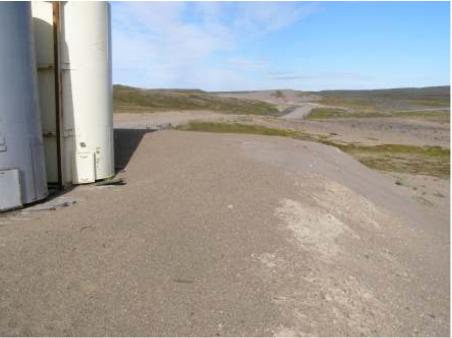
Shows the northeast corner berm with no signs of erosion or deformation.
