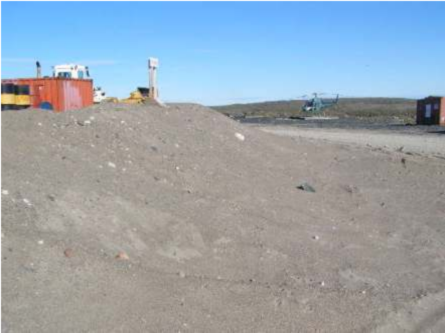
Shows the downstream side of the northern berm, where there is no sign of seepage, sloughing or erosion.
