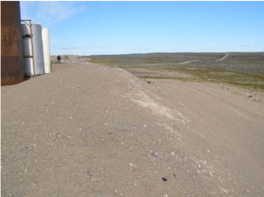
Shows the downstream toe of the east side berm. No signs of erosion, deformation or seepage at this location.
