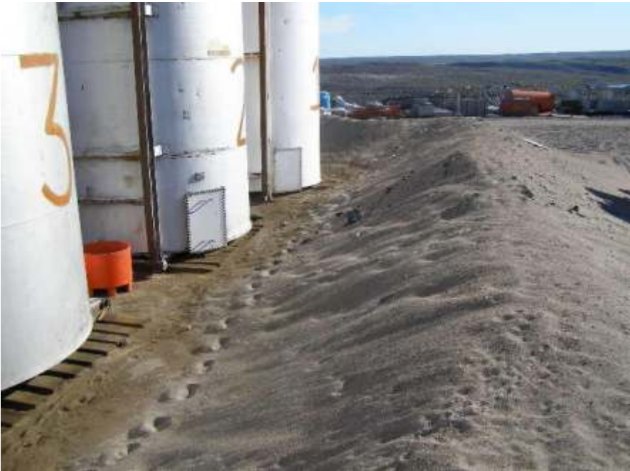
Shows the inside of the sand berm where there’s no sign of standing water.
