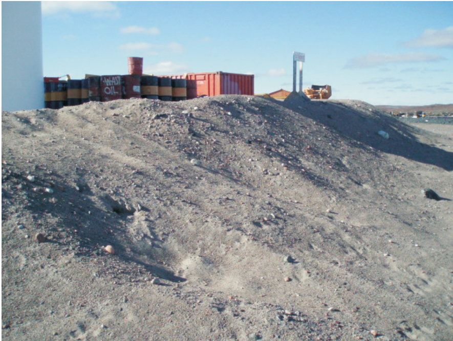
View of the north side berm with no signs of deformation.
