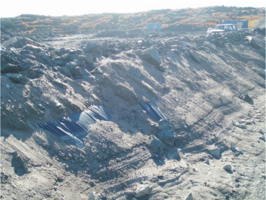
Shows the inside view of the east berm. There are exposures of the liner in approximately three places where the sand cover is fairly thin.
