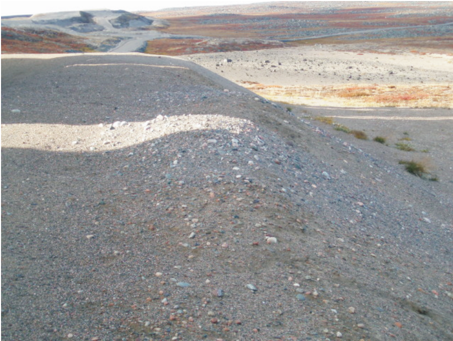
Shows the crest and the downstream side of the berm with no signs of deformation or erosion at the current time.
