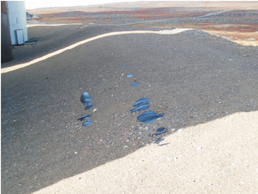
Shows a minor liner exposure on the northern berm.
