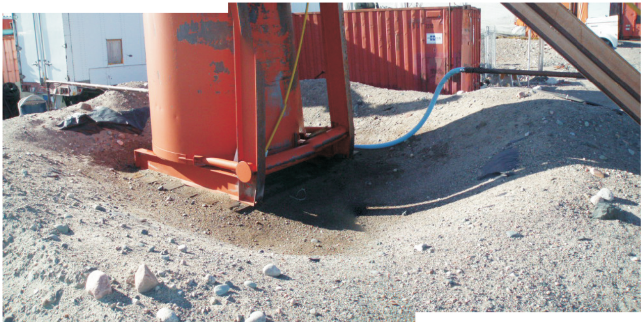
A panoramic of the inside of the containment berm. On the right can be seen one exposure of the liner. On the far left can be seen another directly proximal to the side of the tank.
