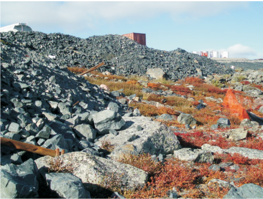
View taken back along the toe looking back towards the Tank Farm. To this distance along the toe, I have not heard or seen any indications of seepage discharging from the toe area.
