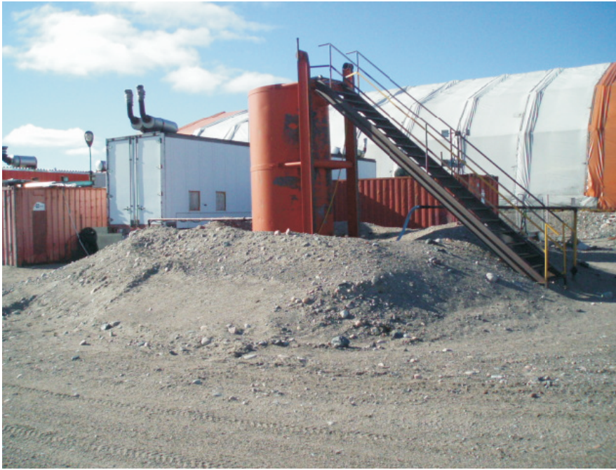
Shows an overall view of the Day Tank Farm. No signs of deformation or erosion of the containment berm.
