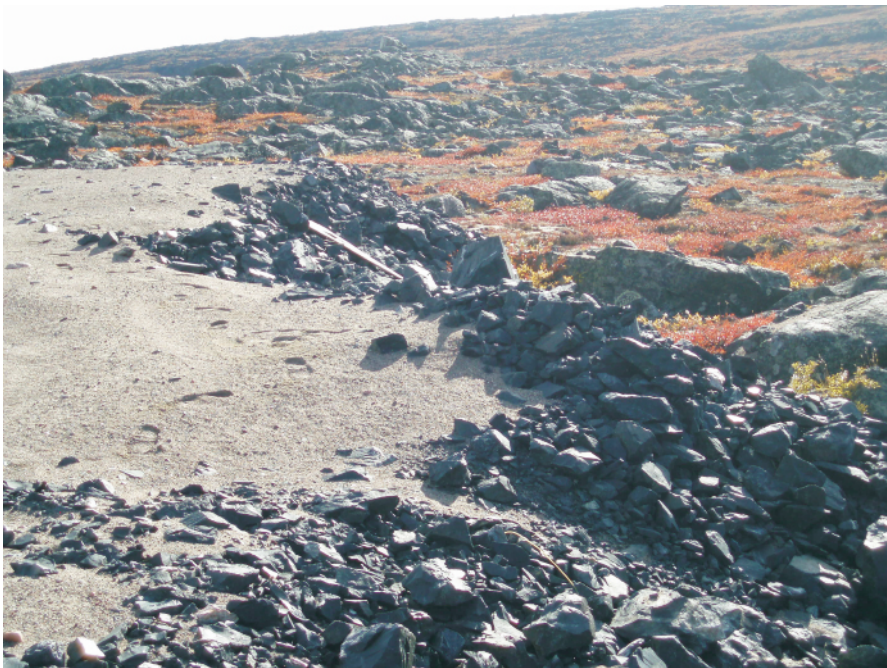
View taken along the southwest corner of the storage pad. No signs of seepage are noted along this edge.
