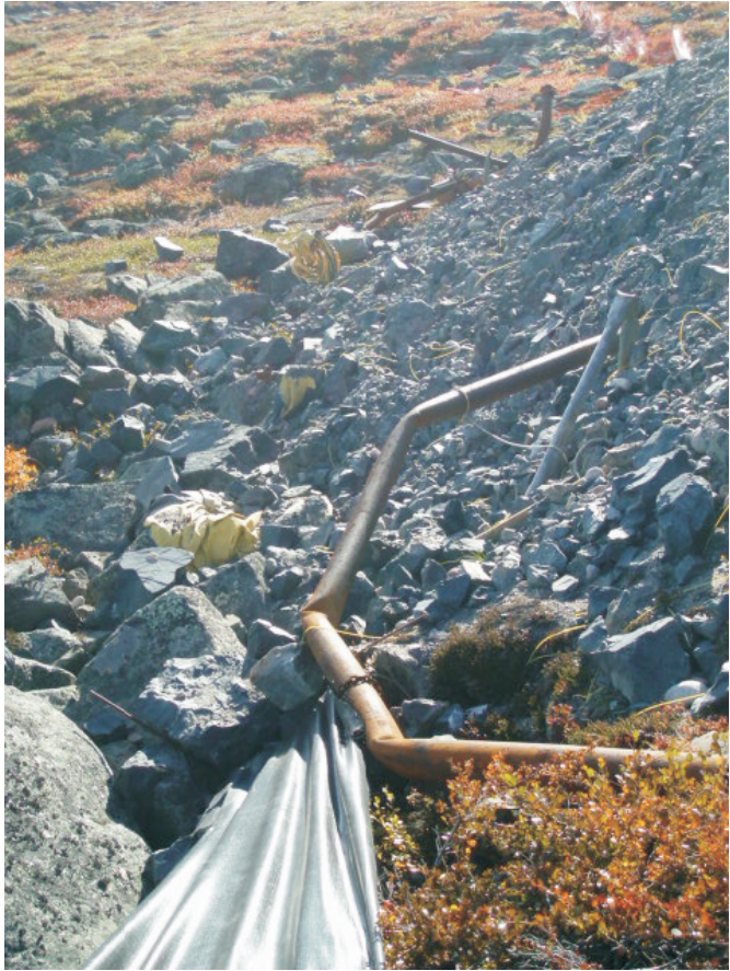
Shows where the fill has overridden the top of the sediment control fence.
