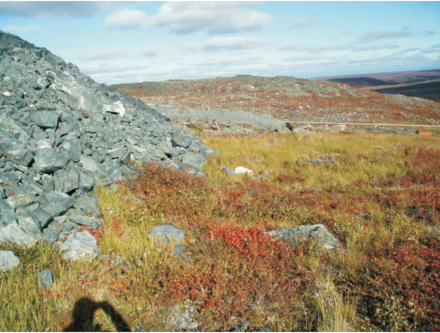
Shows a grassy area located right at the toe of the dump. In this area there is a minor amount of standing water, but no signs of seeping water.
