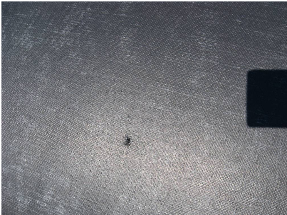
Typical Small Tear in Liner
