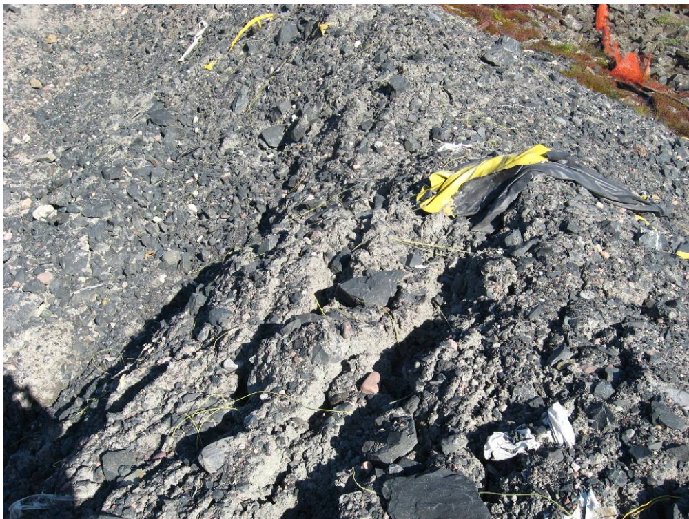
Slump Cracking Downhill Side
