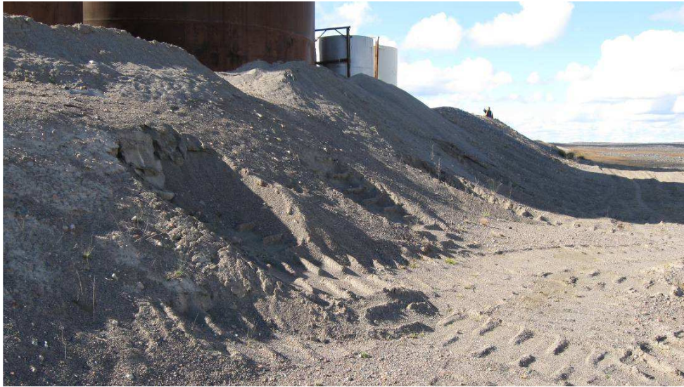
Area of Cut Into Downstream Slope
