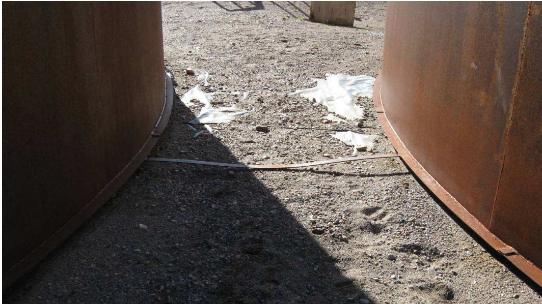
Exposed Liner Between Tanks
