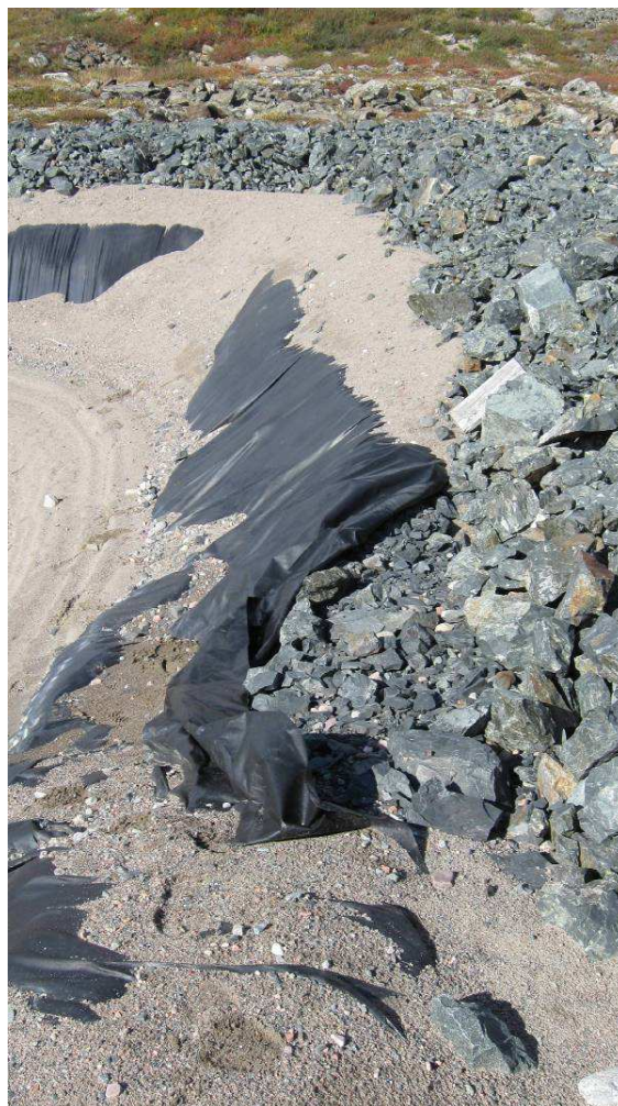
Exposed and Loose End of Liner
