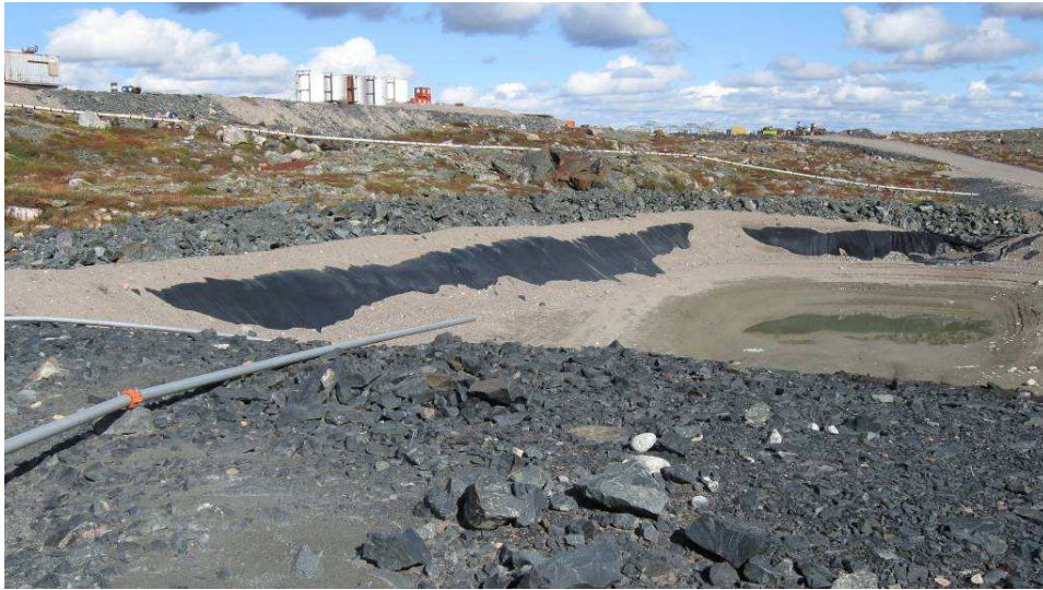
Mine Sump Pit – Exposed Liner
