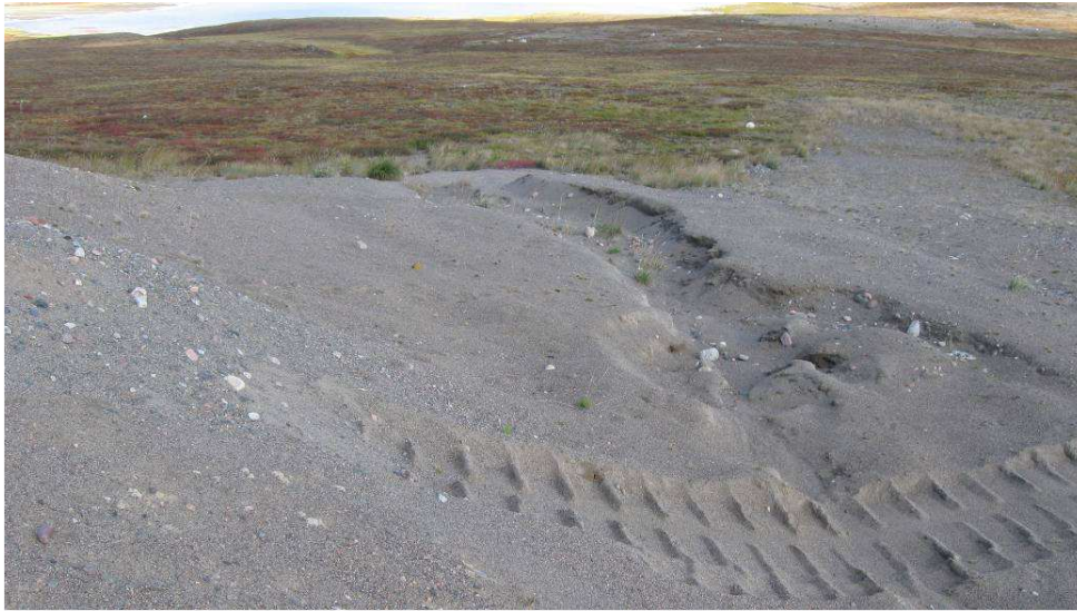
Erosion Gully Near Toe of Embankment S/E Corner
