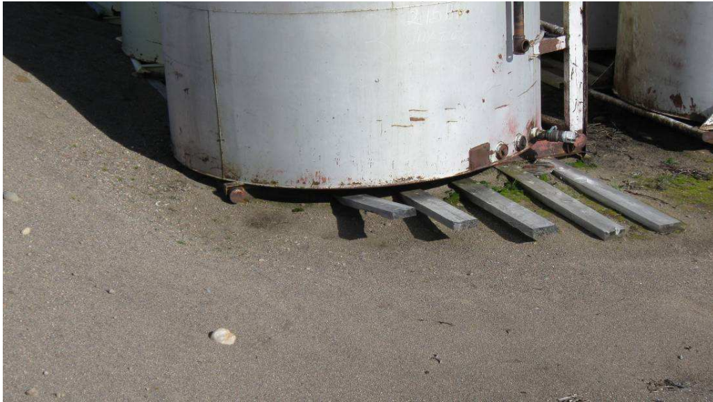
Broken Timber Support
