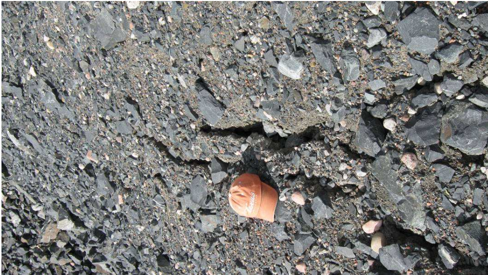
Slump Cracking Downhill Side
