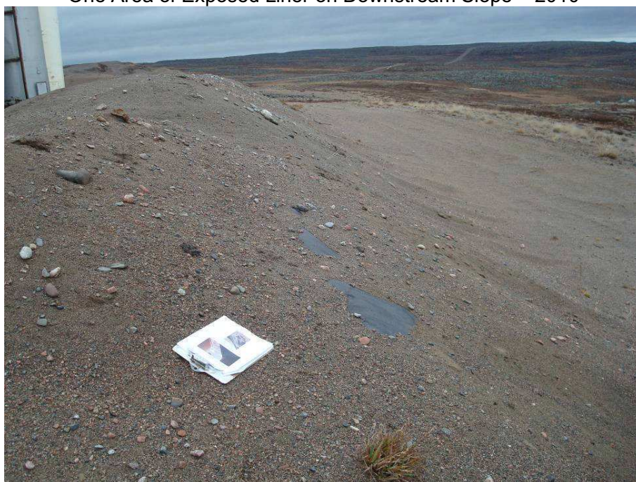
One Area of Exposed Liner on Downstream Slope – 2011
