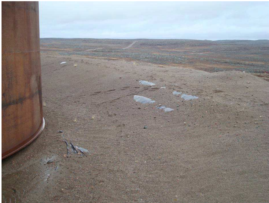
New Area of Exposed Liner – 2011
