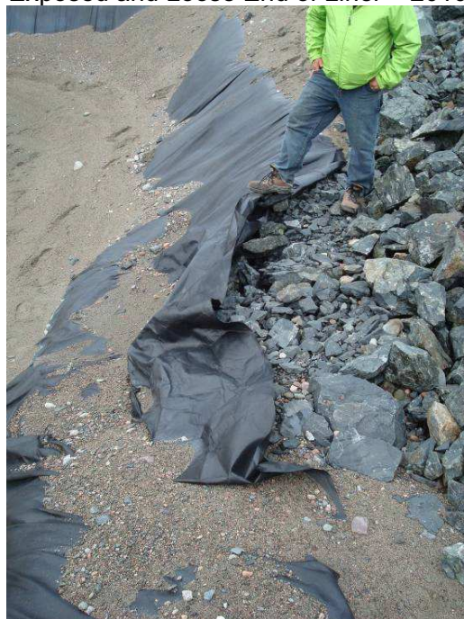
Exposed and Loose End of Liner – 2011
