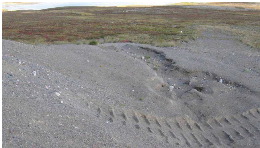
Erosion Gully Near Toe of Berm S/E Corner – 2010
