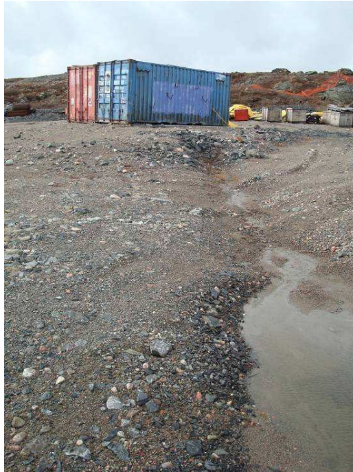
Flowing Surface Water in Small Channel Near Uphill Side of Pad (source of water unknown) – 2011
