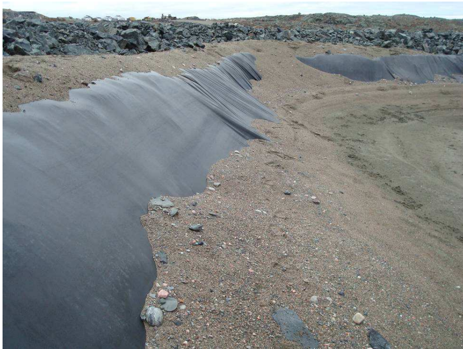
Mine Sump Pit – Exposed Liner – 2011
