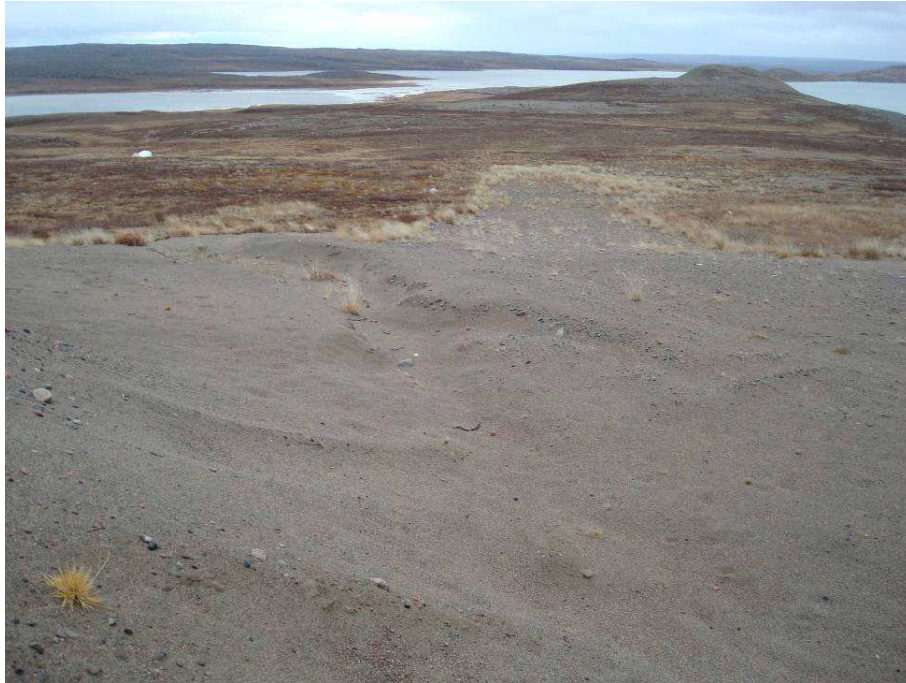
Erosion Gully Near Toe of Berm S/E Corner – 2011
