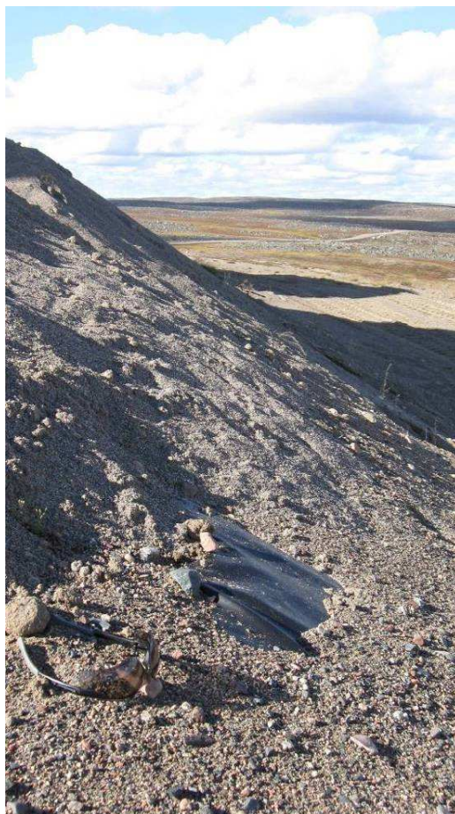
One Area of Exposed Liner on Downstream Slope – 2010
