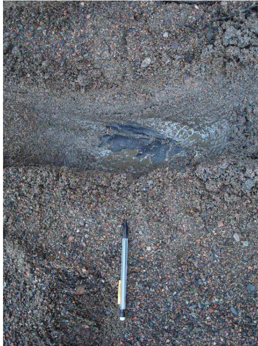
Liner Uncovered At One Location of Containment Area Floor – Appears in Good Shape – 2011
