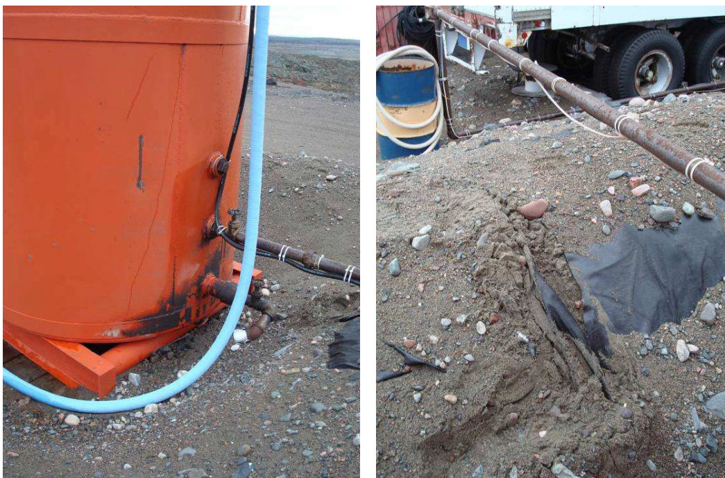
Inside of Berm, West Side with Exposed and Separated Liner – 2011
