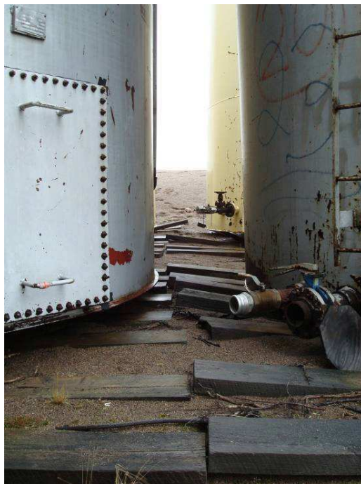
More Broken Timber Tank Supports – 2011
