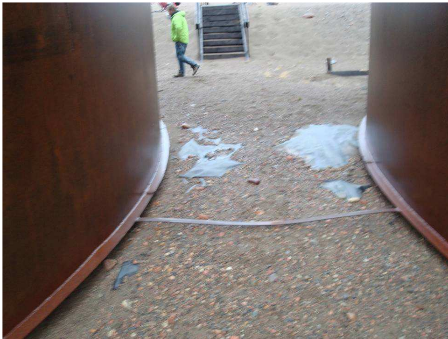
Exposed Liner Between Tanks – 2011
