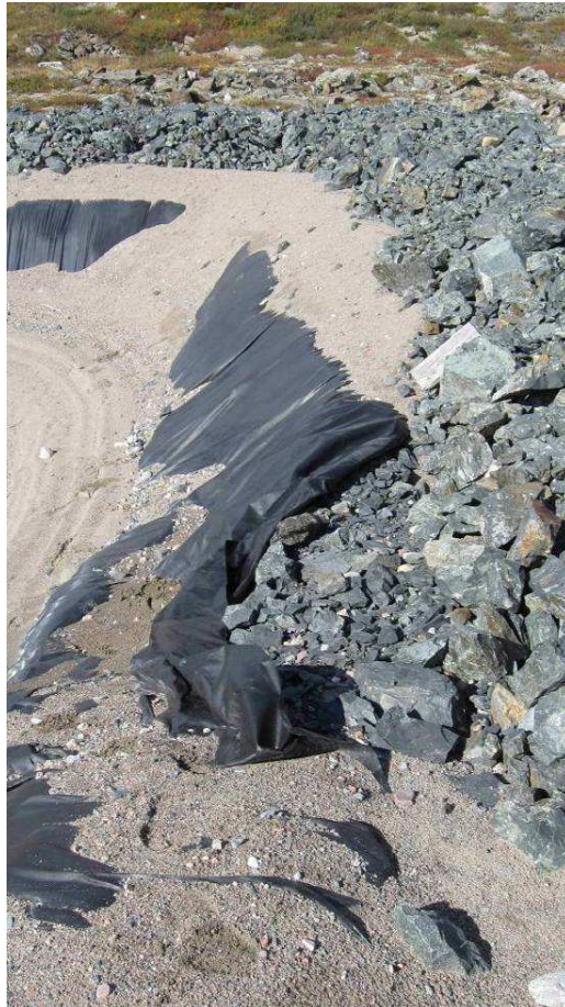
Exposed and Loose End of Liner – 2010
