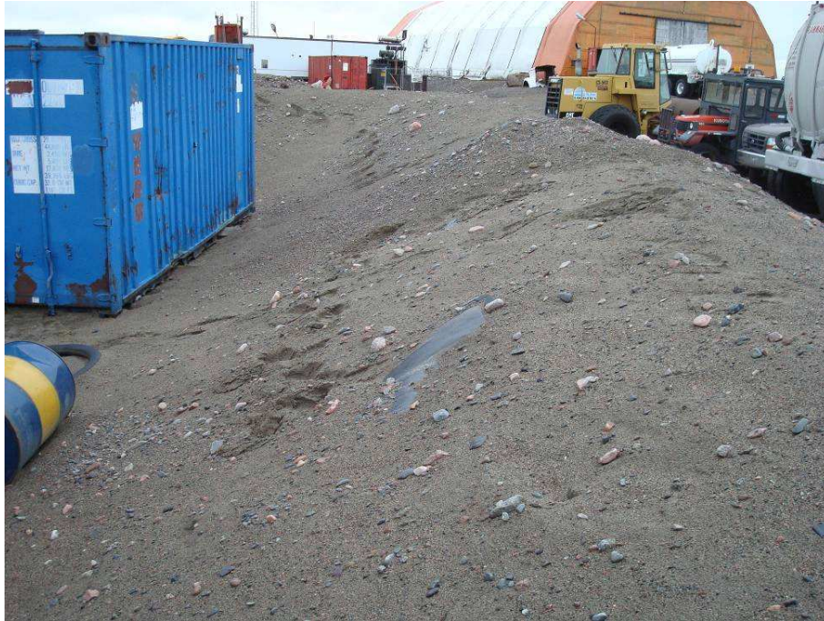
One Area of Exposed Liner – 2011
