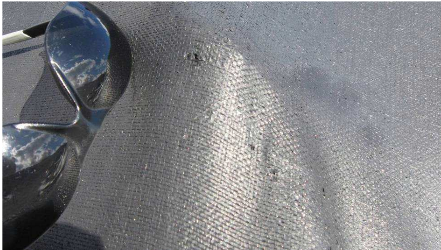
Typical Small Tear in Liner – 2010
