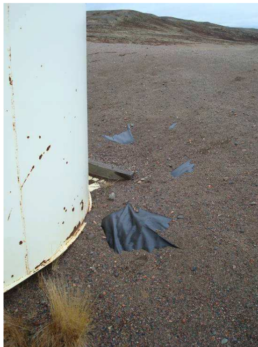
New Area of Exposed Liner – 2011
