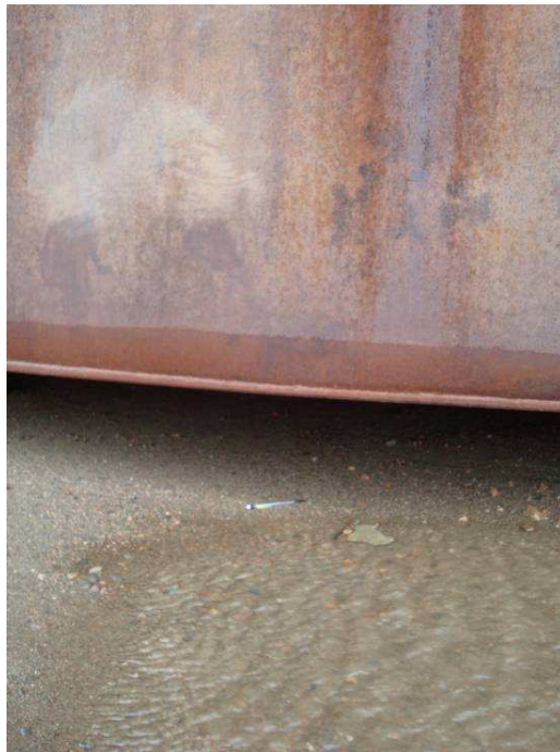
Gap below tank (some contained water) – 2011
