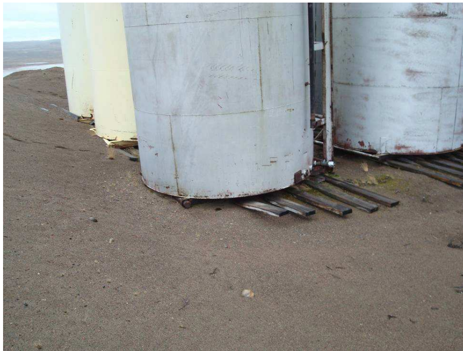
Broken Timber Support – 2011 Another Leaning Tank – 2011
