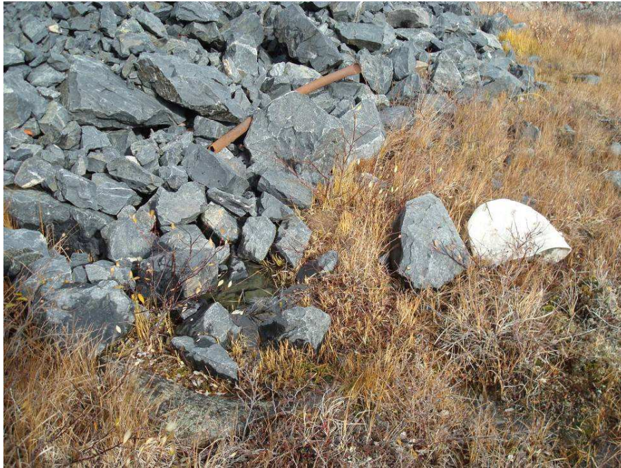
Seepage Noted At One Location, Toe of Pad (est. 1 l/min.) – 2011
