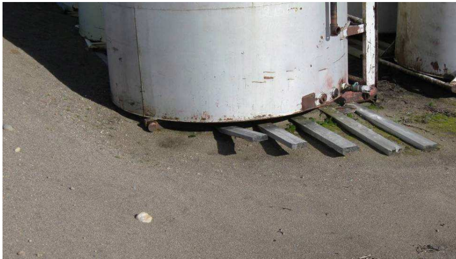
Broken Timber Support – 2010
