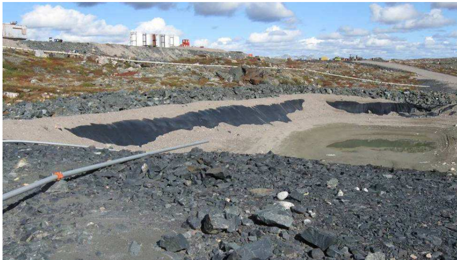
Mine Sump Pit – Exposed Liner – 2010
