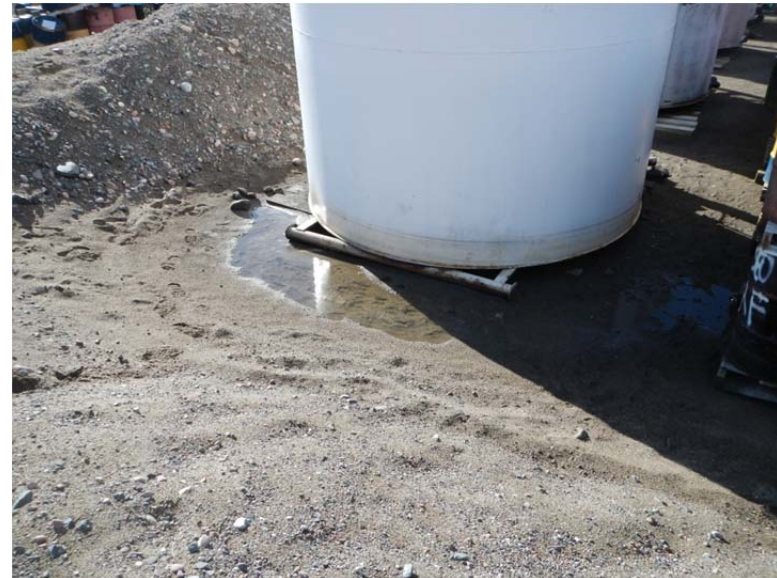
Ulu Tank Farm Ponding Water
