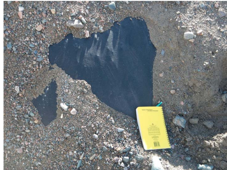
Ulu Tank Farm Exposed Liner
