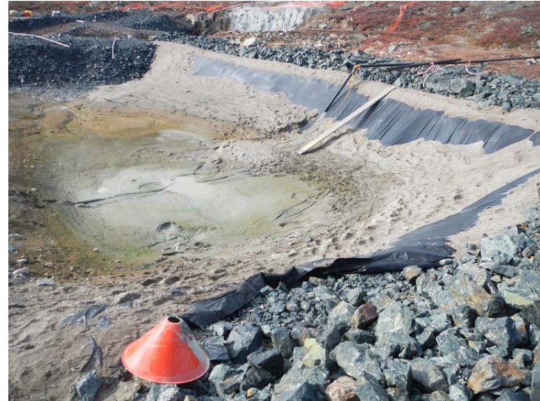
Ulu Mine Sump Exposed Liner and leading edge
