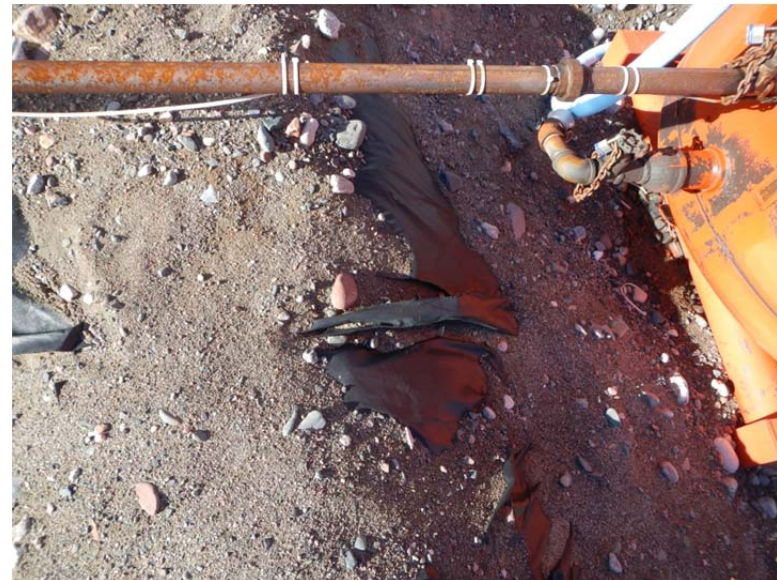
Ulu Day Tank Damaged Liner
