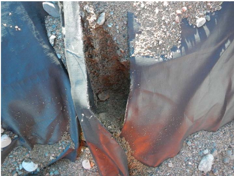
Ulu Day Tank exposed and damaged liner (closer view)
