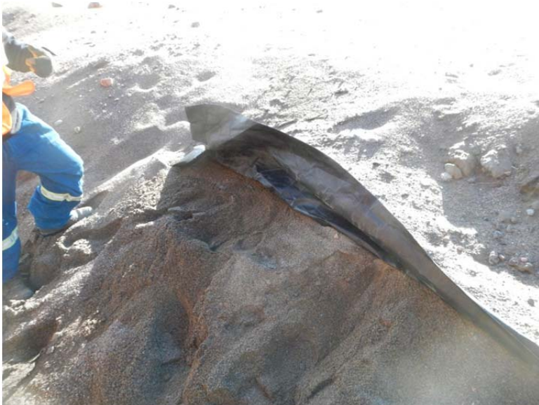
Ulu Tank Farm Exposed Liner
