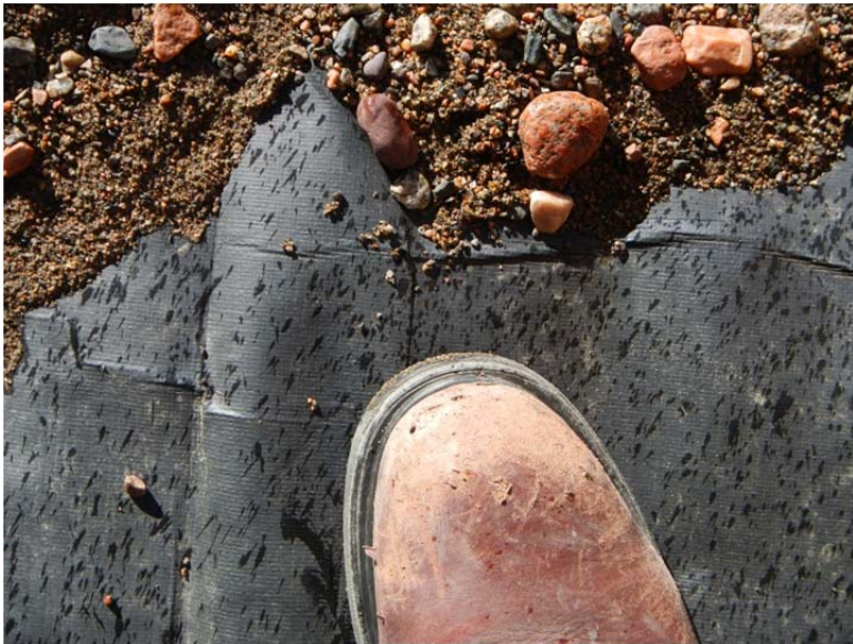
Ulu Tank Farm Exposed Liner
