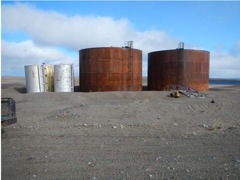
Camp 3 Tank Farm and the leaning empty fuel tank
