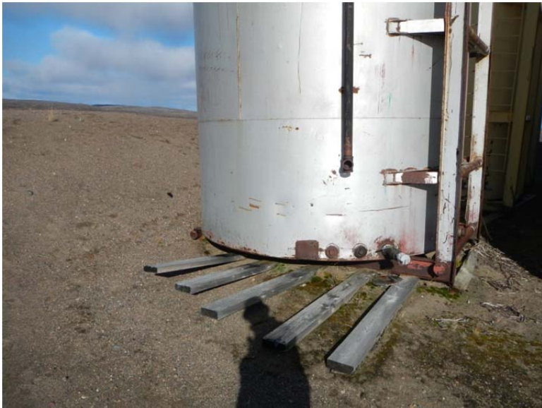
Camp 3 Tank Farm Broken Cribbing
