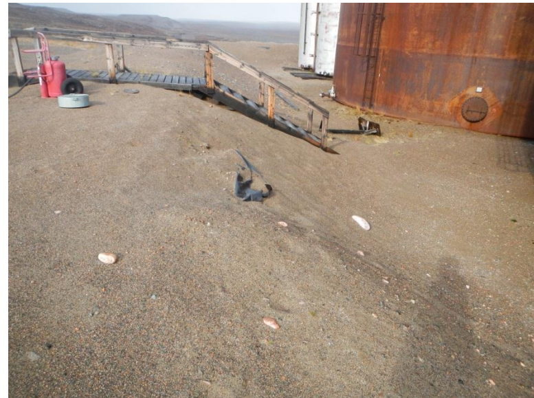
Ulu Camp 2 tank farm, view of exposed liner
