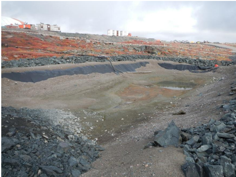
Ulu mine sump, view of exposed liner
