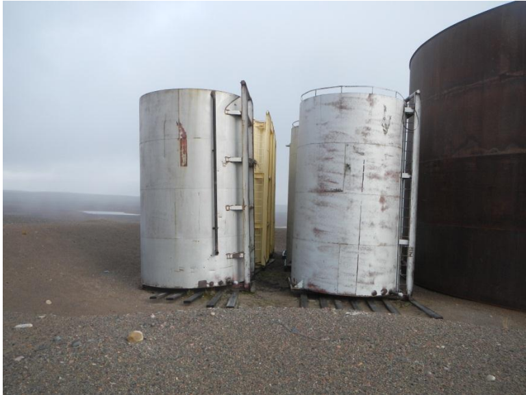
Ulu Camp 3 tank farm, view of leaning fuel tank
