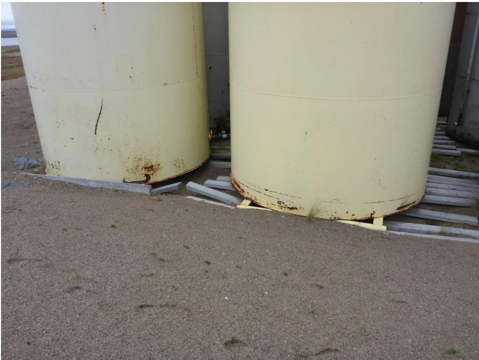
Photo 10: Close up view of the broken cribbing underneath the leaning tanks.
