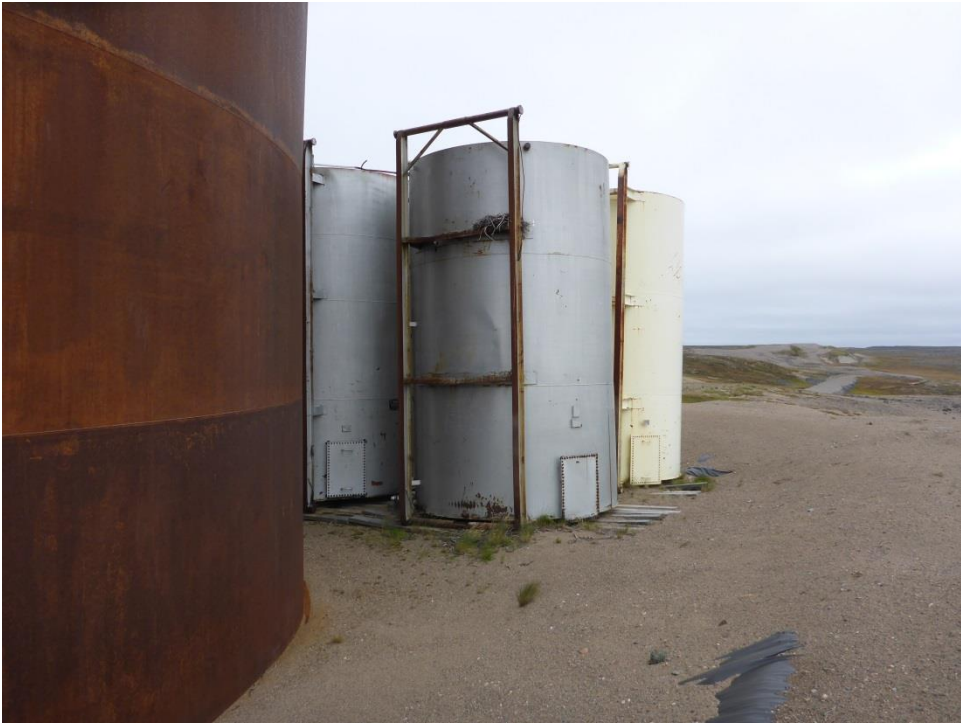
Photo 7: Looking north at the leaning tanks at the back of the Camp 3 fuel tank farm.
