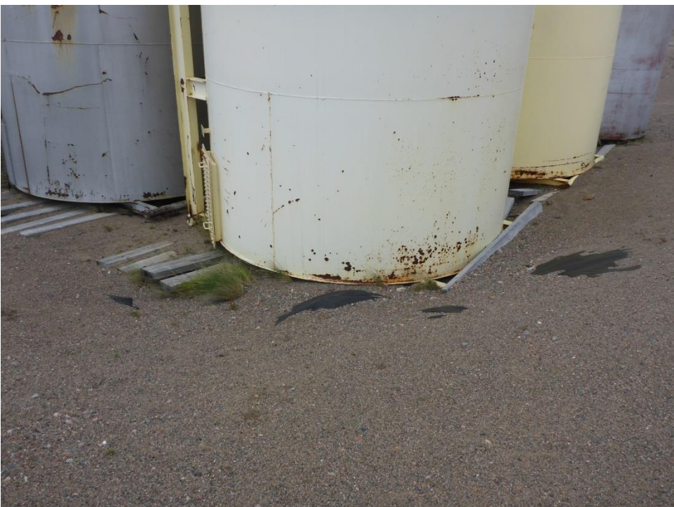
Photo 8: Close up view of the broken cribbing underneath the leaning tanks.
