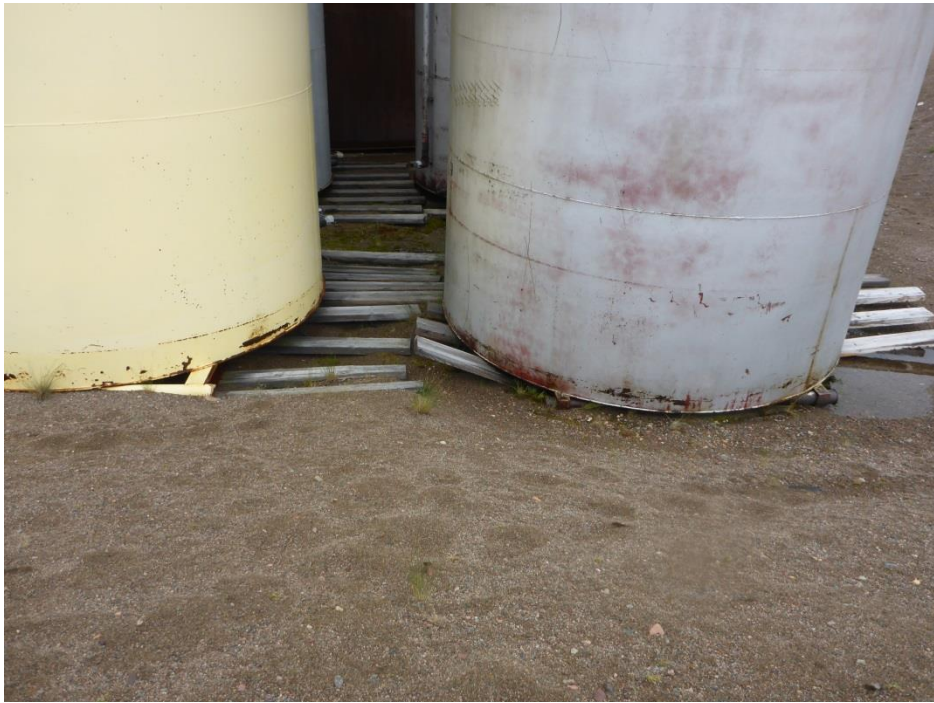
Photo 2: Close up view of the broken cribbing underneath the tank.
