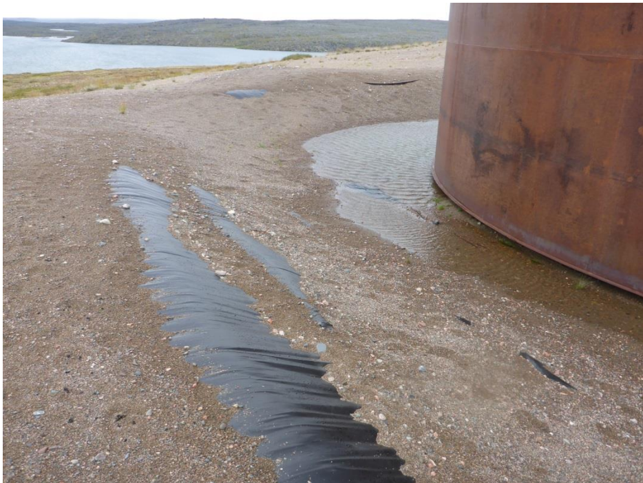
Photo 5: Close up view of the exposed liner and water ponding underneath the large tanks in Camp 3 fuel tank farm.
