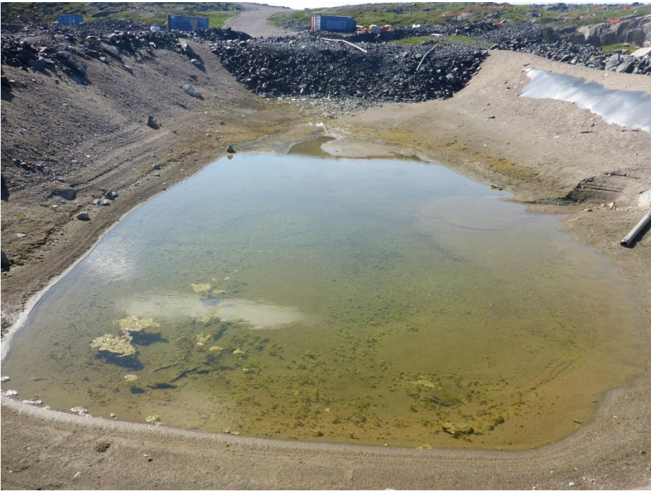
Photo 8: Looking west at the mine sump. Note the exposed liner on the north bank.
