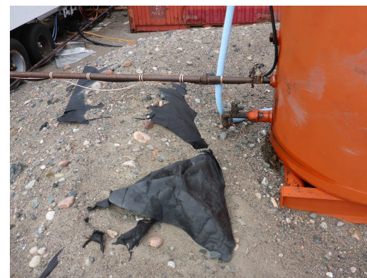
Photo 17: Looking at the exposed and damaged liner at the south side of the day use tank containment berm.
