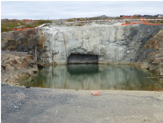
Photo 21: Looking at the submerged bulkhead of the mine portal.
