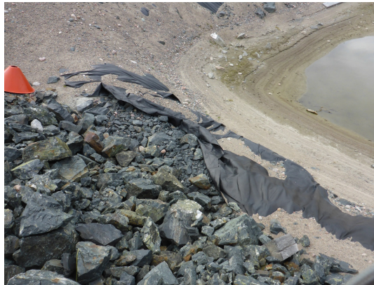
Photo 8: Looking at the northern edge of the exposed liner in the mine sump.
