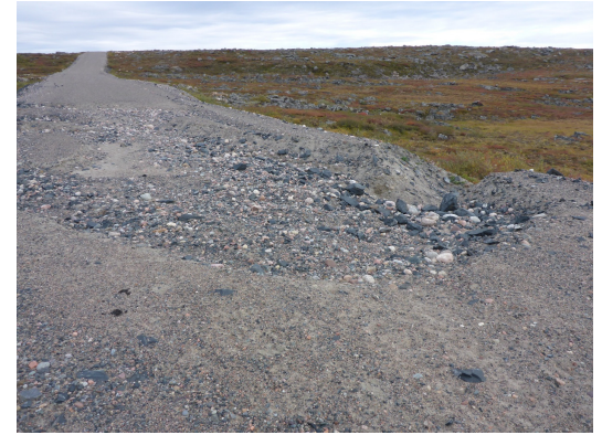
Photo 20: Looking at one of the large erosion gullies across the access road between the airstrip and Camp 3.
