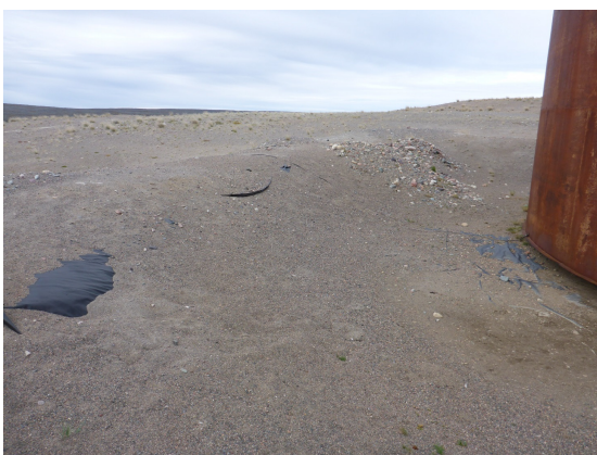
Photo 5: Looking at the exposed and damaged liner at the southeast corner of the tank farm.
