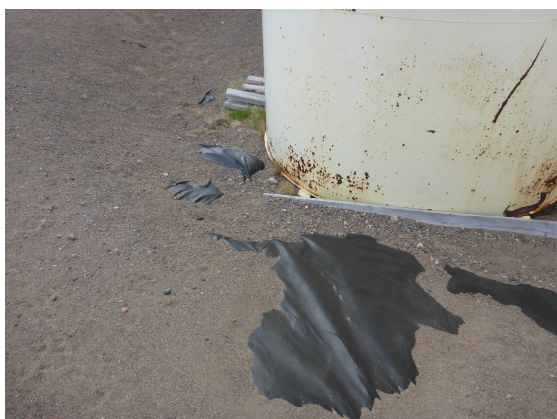
Photo 4: Looking at the exposed and damaged liner at the northeast corner of the tank farm.
