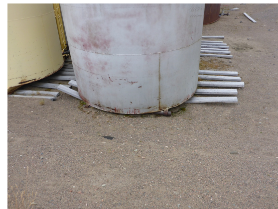
Photo 3: At the broken wooden cribbing at the base of the leaning tank.
