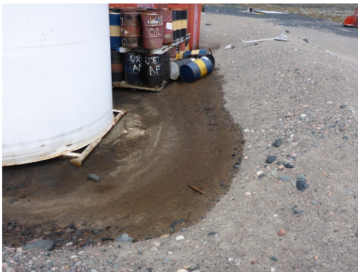
Photo 13: Looking at the south side of the containment berm. Note the high water mark.
