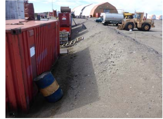
Photo 14: Looking at the west side of the containment berm with the exposed liner.
