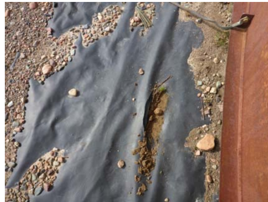
Photo 5: Looking at the exposed and damaged liner between the tanks.
