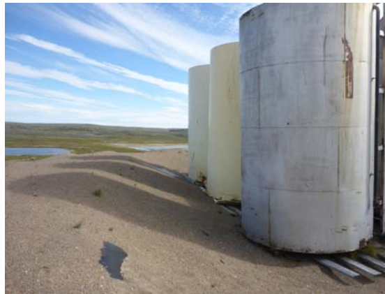
Photo 2: Looking southeast at one of the leaning 53 thousand litres tank.
