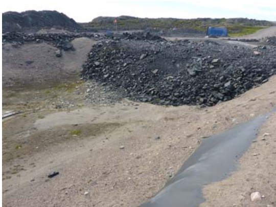
Photo 7: Looking southwest at the exposed liner in the mine sump
