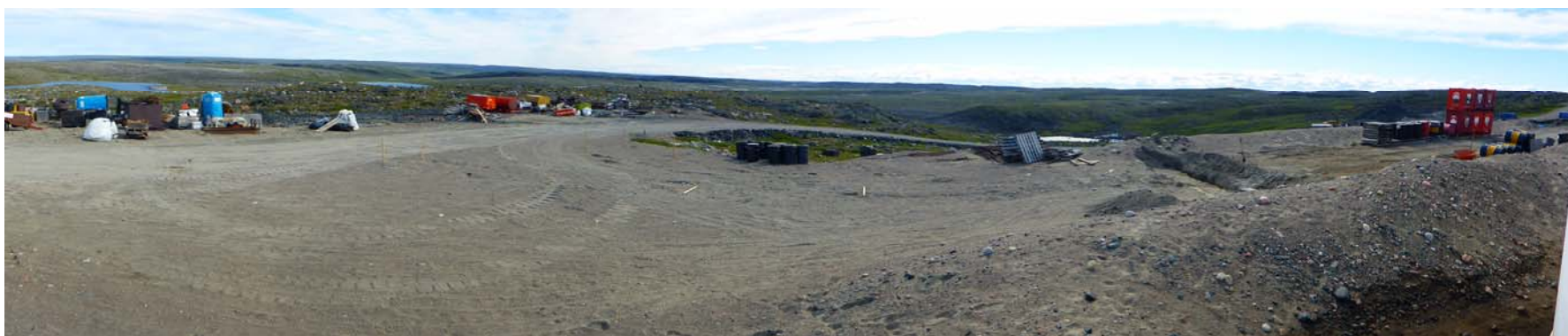
Photo 21: Panoramic south looking view at the fuel transfer area mitigative work, including exposing the edge of the underlaying liner and start of berm construction.
