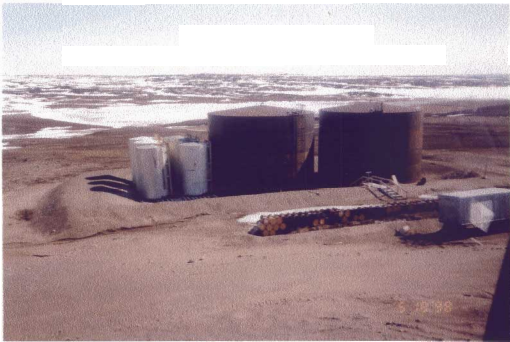
Photo 4 Ulu Project Camp 3 Fuel tank farm looking from the west. Two 350,000 usg tanks and six 14,000 usg tanks to the left Off loading apron in foreground with fuel drum storage.
