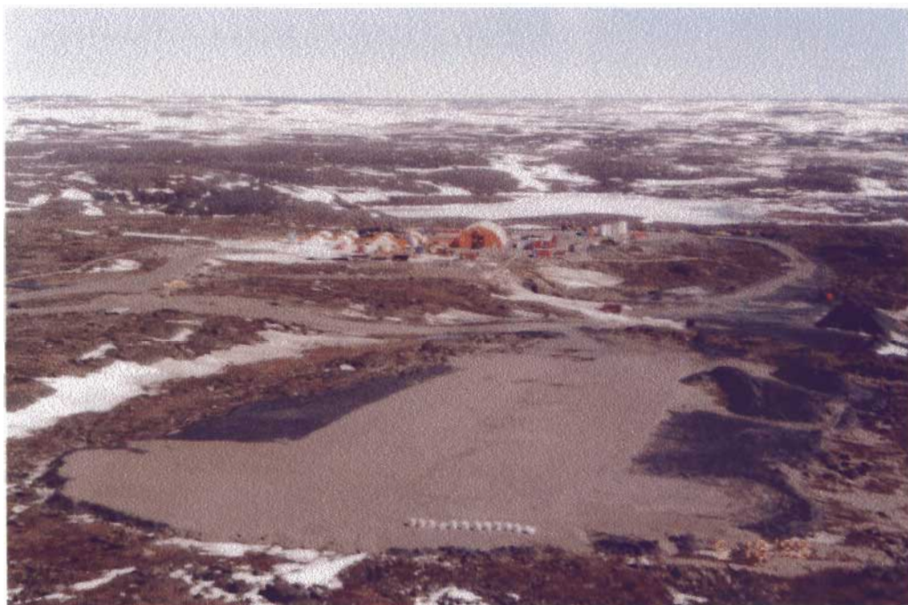
Photo 2 Ulu Project Camp looking from the south. Incomplete ore storage pad in foreground, weatherhaven shop and camp in centre with Ulu Lake in the background.
