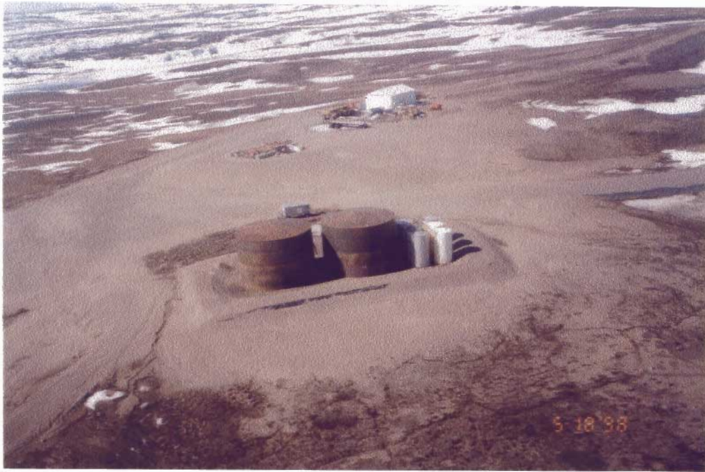
Photo 3 Ulu Project Camp 3 at Reno Lake looking from the east. Fuel tank farm in foreground. Steel clad shop and equipment storage above. Road accesses to Ulu Camp on right, explosives magazine above right.
