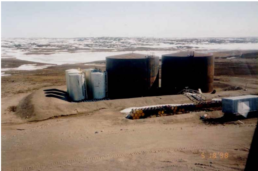
Photo 4: Ulu Project Camp Fuel tank farm looking from the west. Two 350,000 usg tanks and six 14,000 usg tanks to the left of loading apron in foreground with fuel drum storage.
