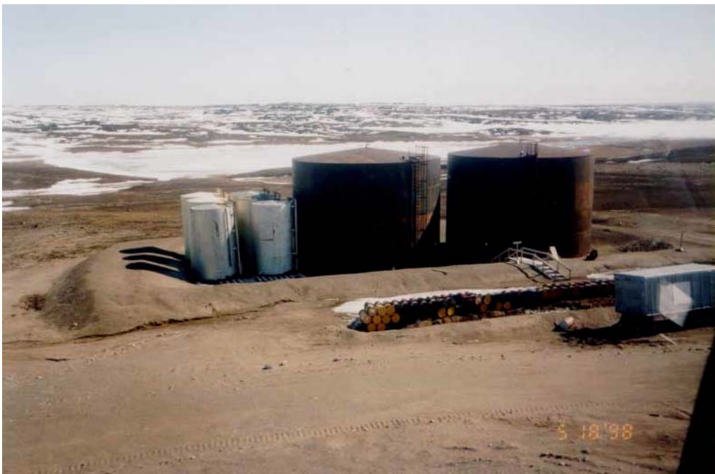
Photo 4 Ulu Project Camp3 Fuel tank farm looking from the west. Two 350,000 usg tanks and six 14,000 usg tanks to the left of loading apron in foreground with fuel drum storage.
