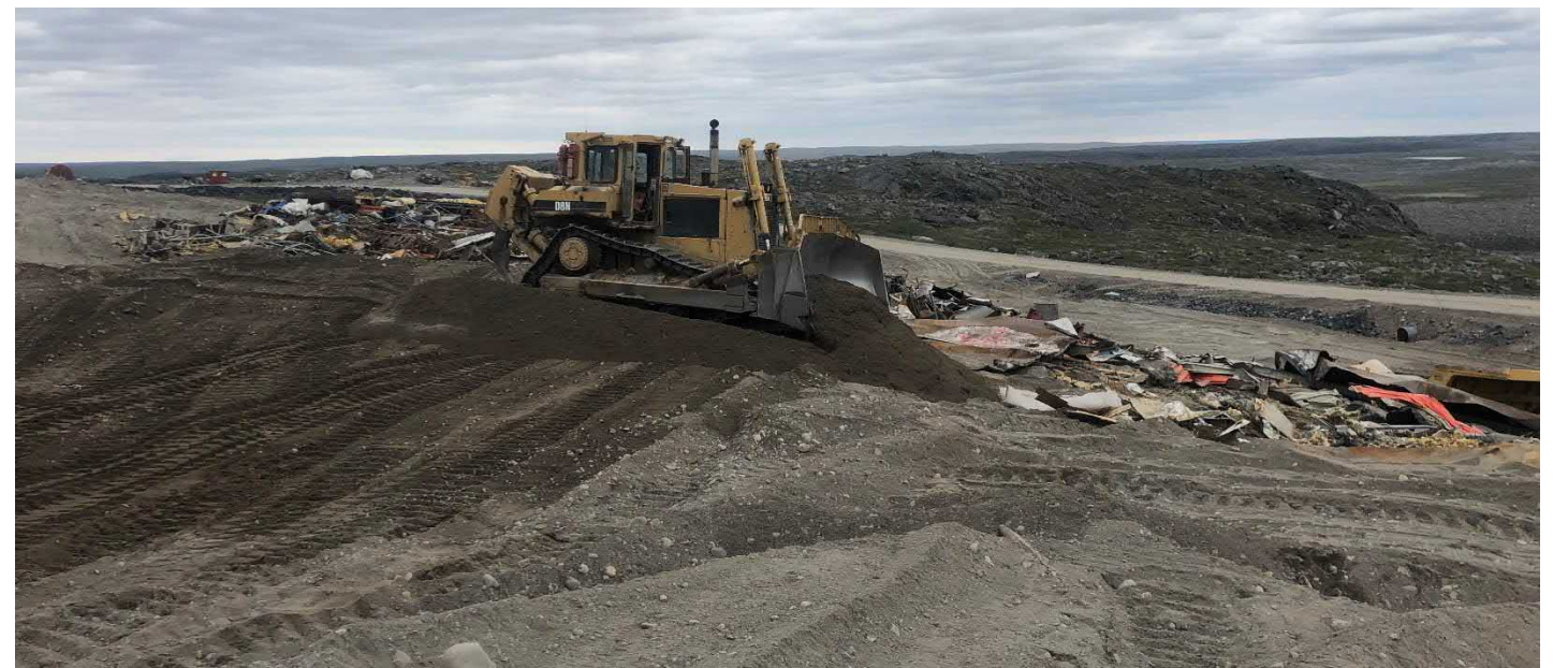
Placing esker sand on August 9, 2021
