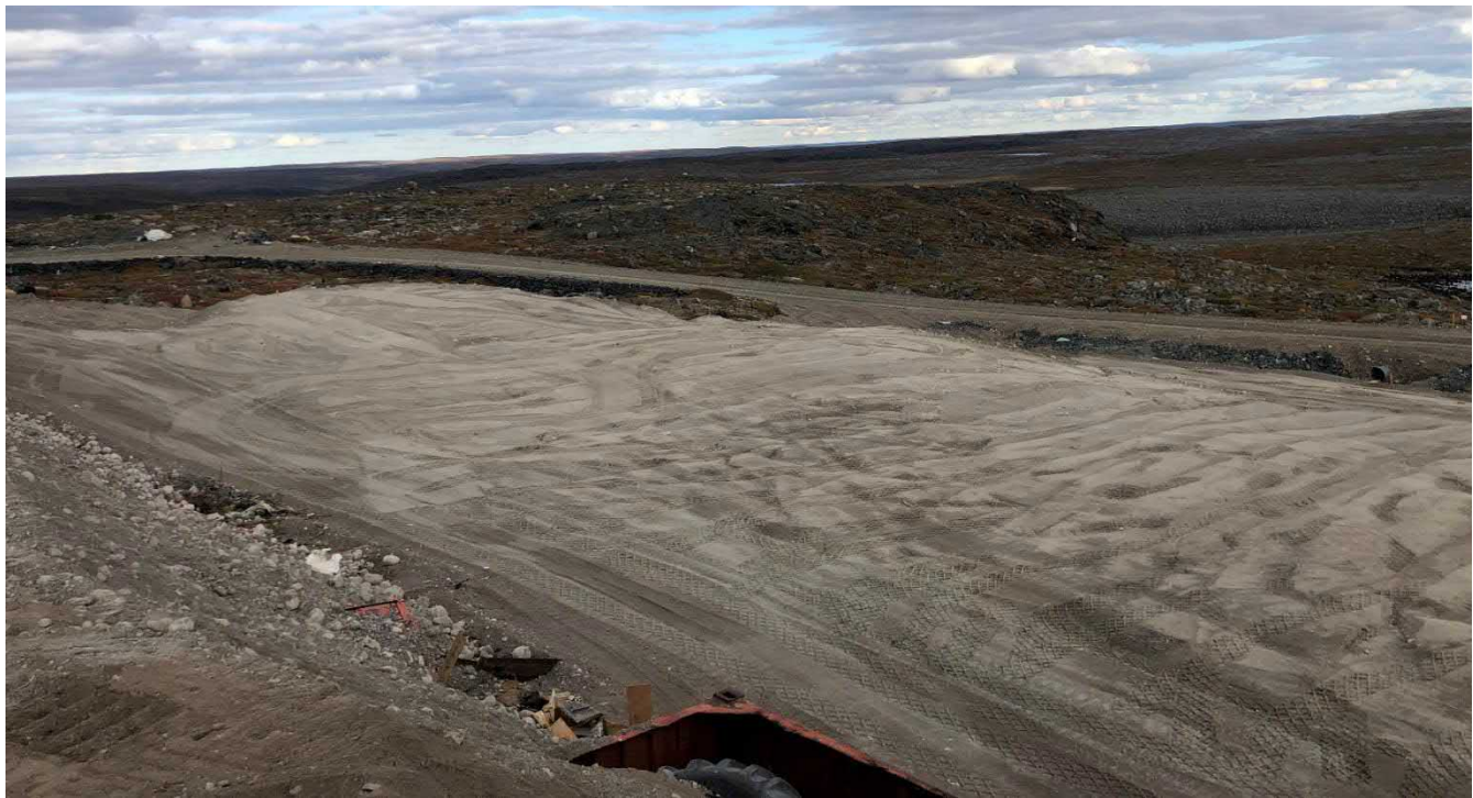
The north side of the site facing southeast with interim cover compaction on August 19, 2021
