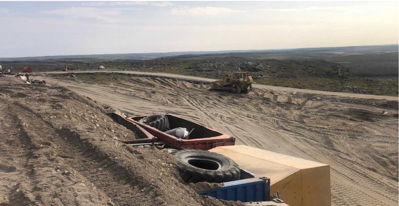
Esker sand placed over waste. August 13, 2021
