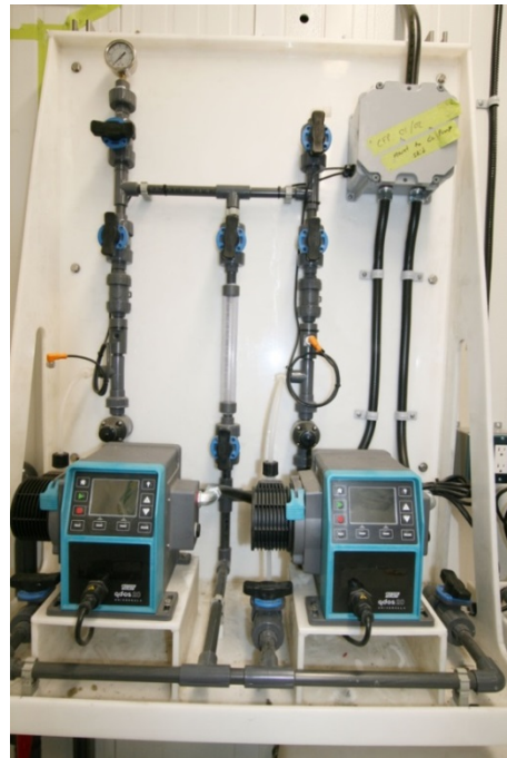
Figure 27 Peristaltic chlorine pumps
