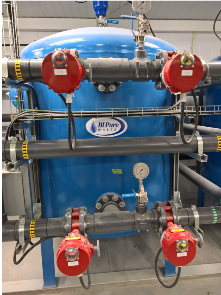
Figure 12 Contact tank, followed by 4 filters containing sand media
