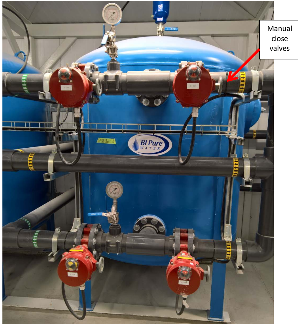
Figure 14 Media filter with fluid direction labels
