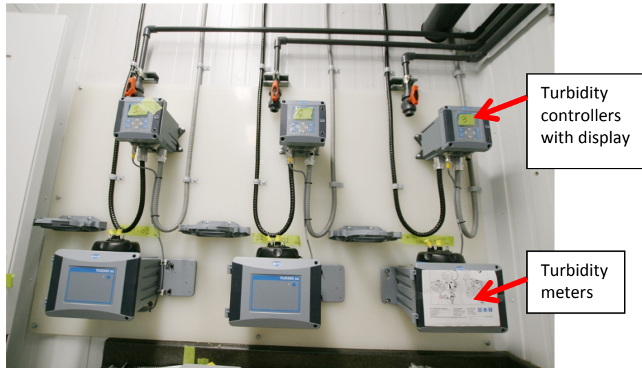
Figure 32 Turbidity meters -01, -02, -03 in the computer room
