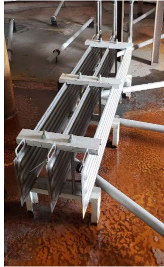
Figure 47 Backwash tank heat exchangers
