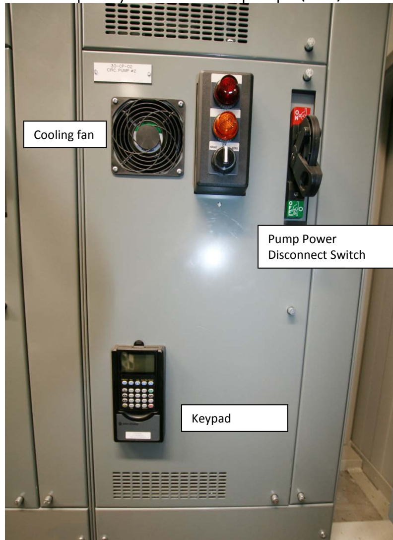
Figure 49 Panel housing the VFD (variable frequency drive) for each pump, in the MCC room
