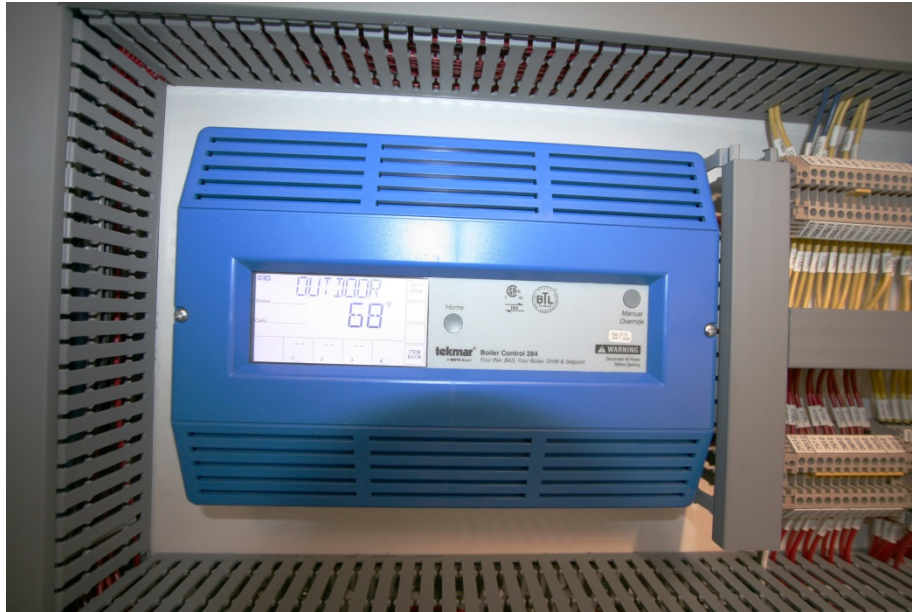
Figure 40 Tekmar controller inside the boiler control panel
