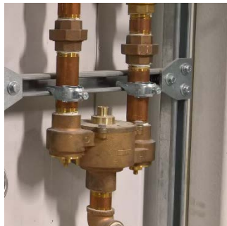
Figure 25: Mixing valve
