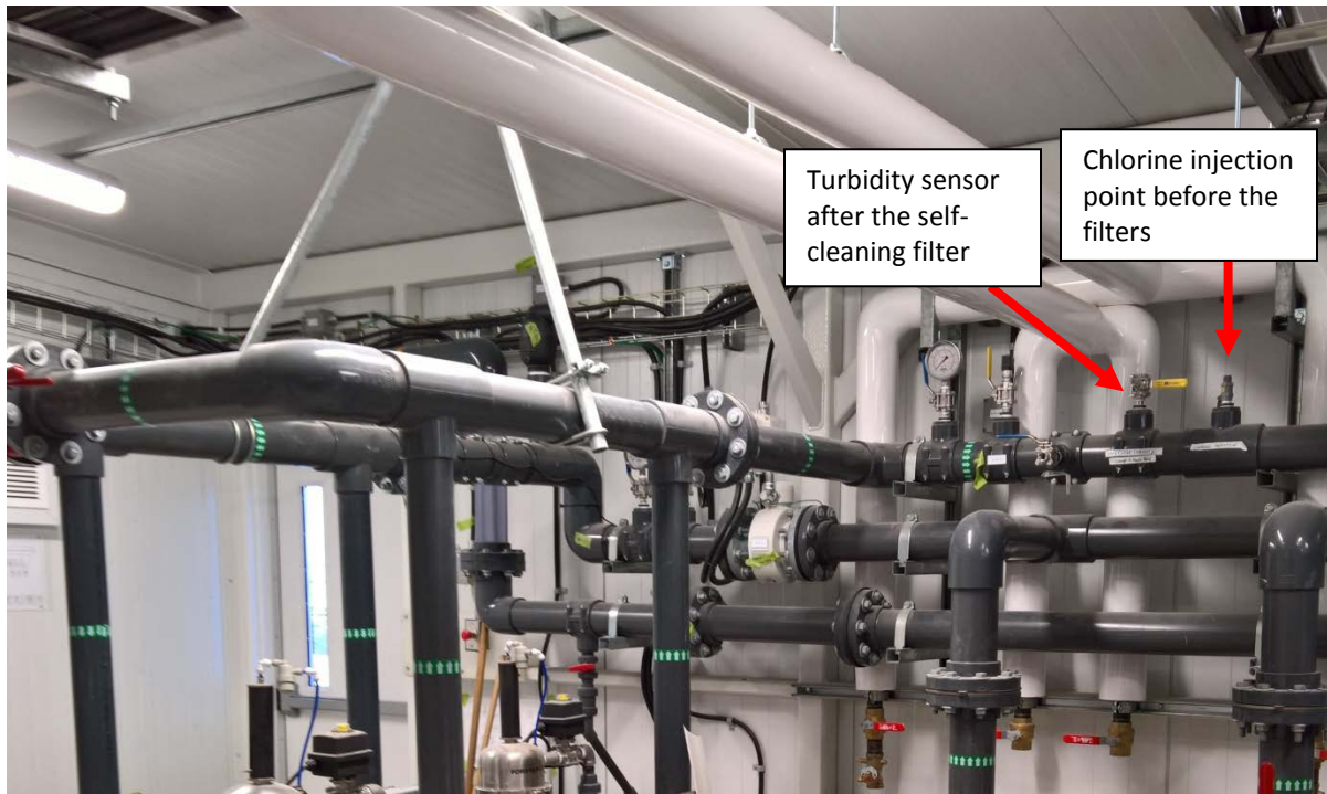
Figure 29 Chlorine injection point preceding the filters
