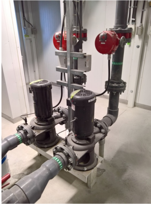
Figure 34 Truckfill pumps
