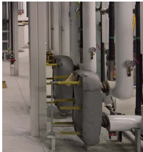
Figure 46 Treated water tank heat exchangers
