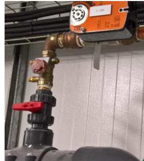
Figure 26: Domestic water balancing valve
