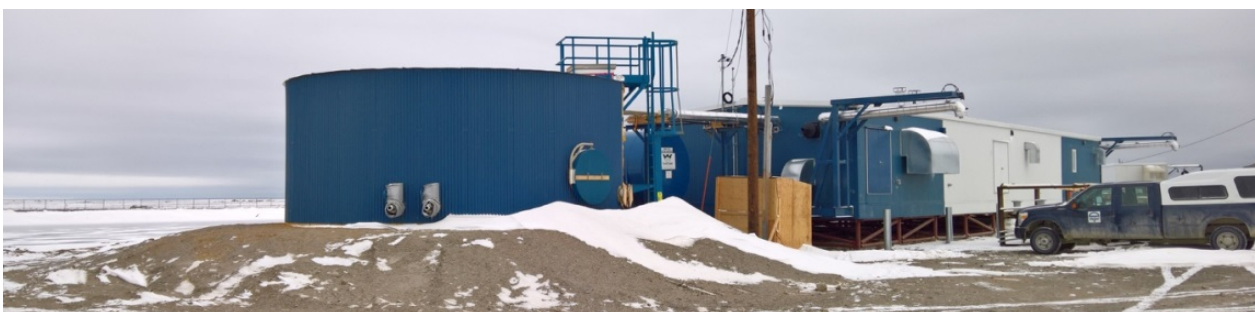
Figure 36 Backwash (process wastewater storage) tank with exterior fuel tank beside it
