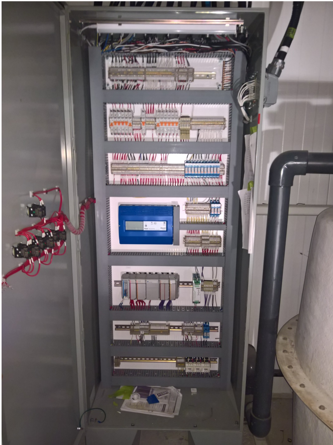
Figure 54 Interior of Boiler Control Panel
