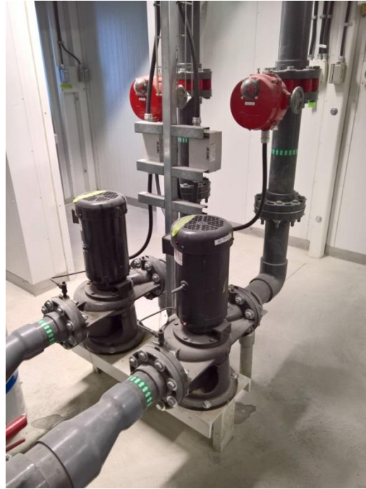
Figure 34 Truckfill pumps
