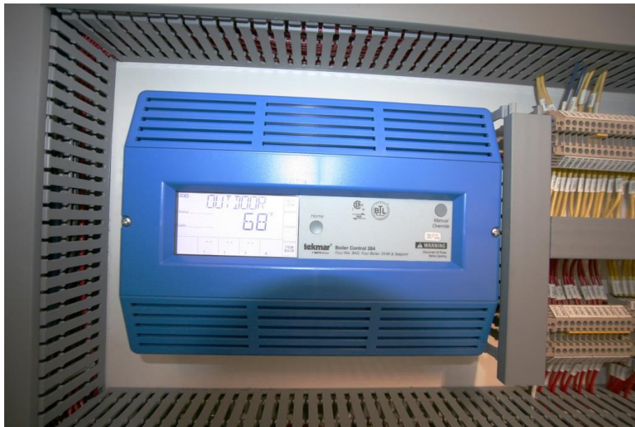
Figure 40 Tekmar controller inside the boiler control panel
