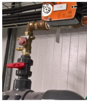
Figure 26: Domestic water balancing valve
