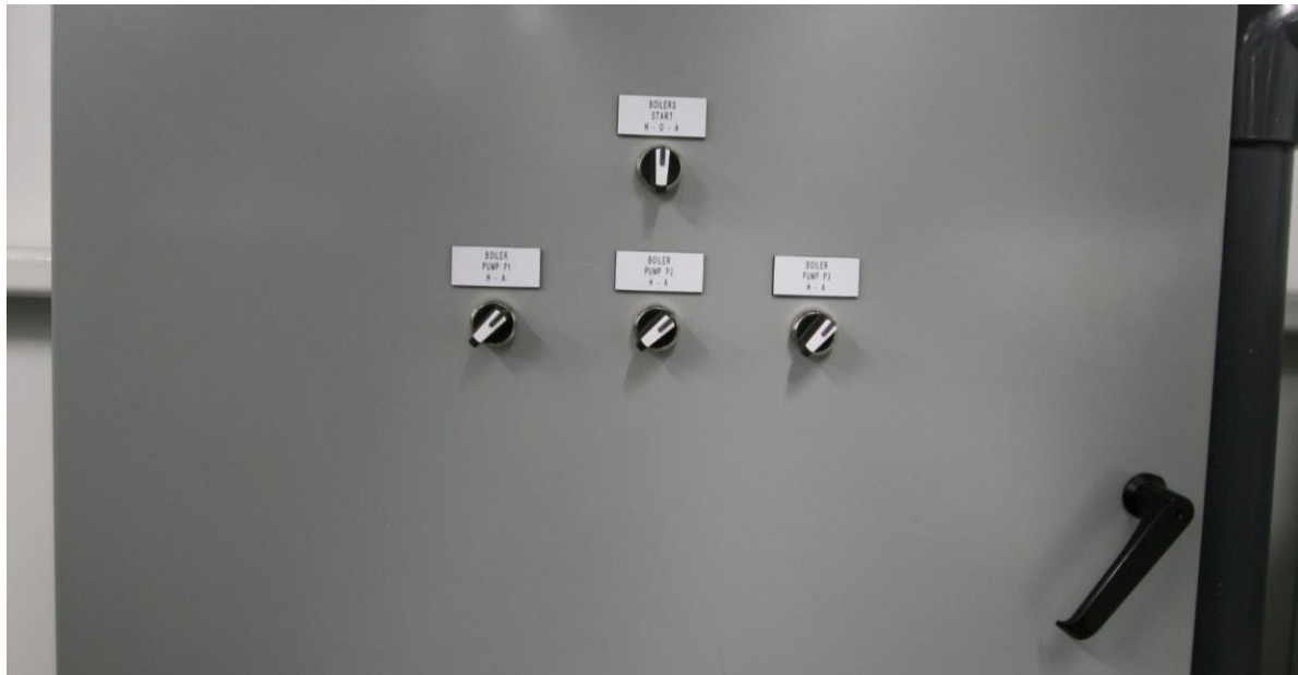
Figure 53 Boiler Control Panel C
