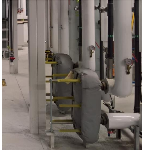
Figure 46 Treated water tank heat exchangers
