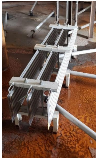
Figure 47 Backwash tank heat exchangers inside the tank
