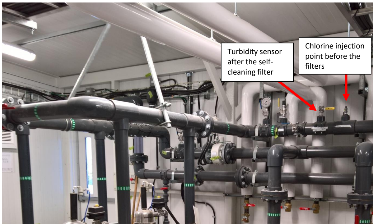
Figure 29 Chlorine injection point preceding the filters
