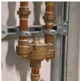
Figure 25: Mixing valve
