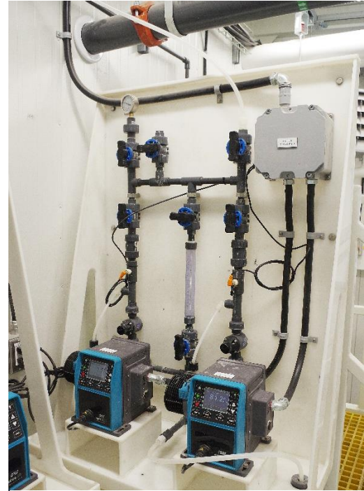
Figure 27 Final disinfection pumps 20-CP-03 and 20-CP-04
