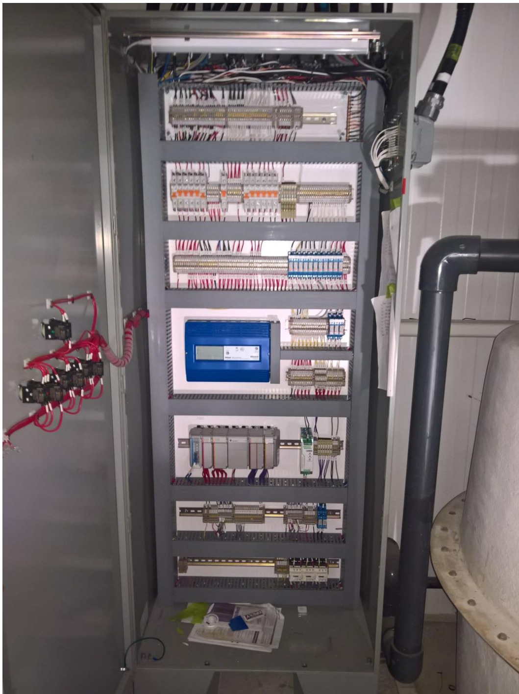
Figure 54 Interior of Boiler Control Panel
