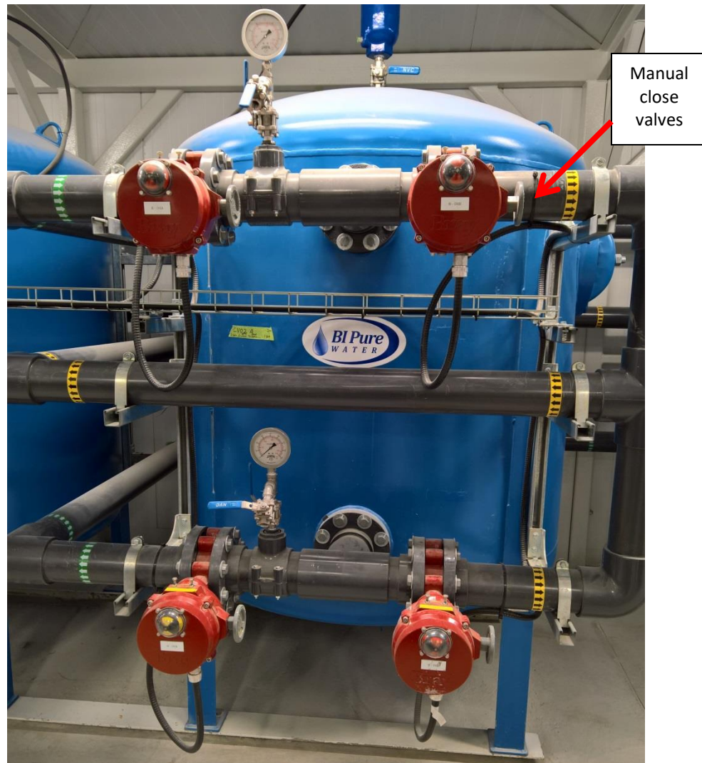
Figure 14 Media filter with fluid direction labels
