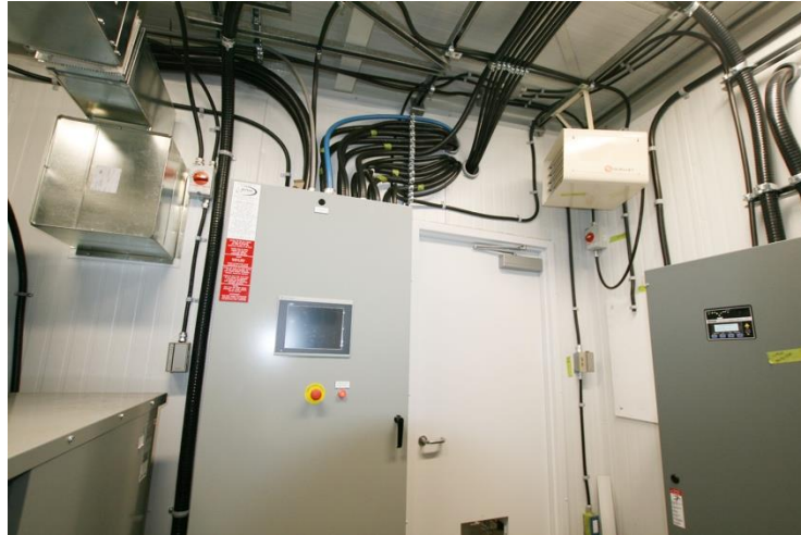
Figure 6 the main control panel inside the Motor Control Centre (MCC room). Power Auto Transfer Switch on the right
