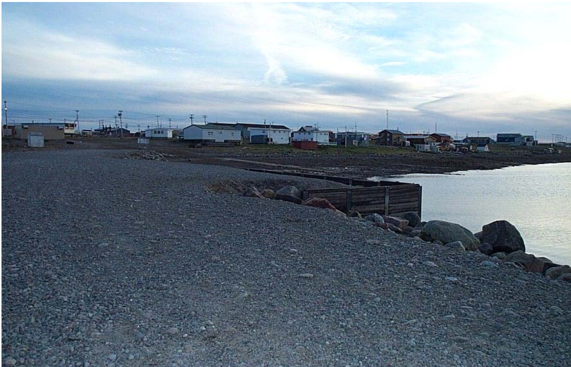
View of Arviat marine bulk-fuel resupply facility (~ 13 meters width x 100 m length) on west face of Breakwater / Wharf. Photo 2-2
