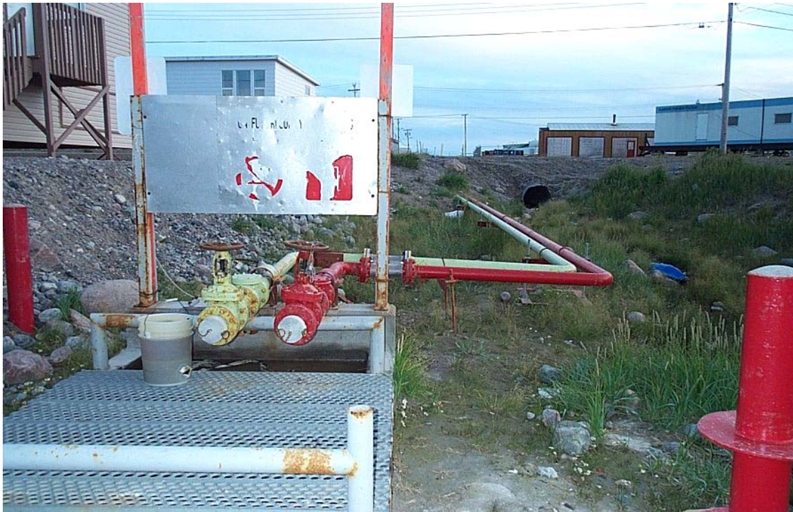
View of pipe header on east side of access road to marine bulk fuel-resupply facility. Photo 5-4
