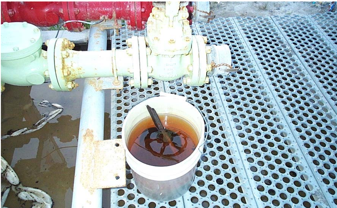
Lack of Best Practices at fuel-resupply facility (20 litre pail with no lid, unknown contents, oily appearance) without drip tray on open-metal grate above bare ground beneath pipe header. Photo 5-5
