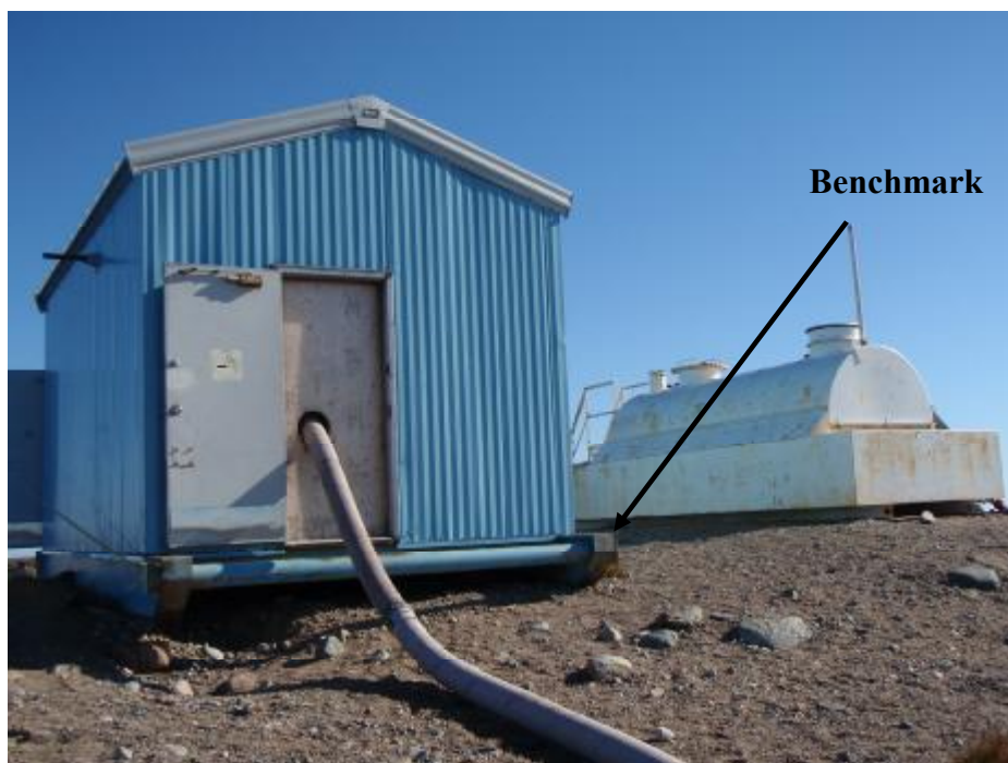
ARV-7 - Water level in Wolf River. Notes: Survey water level from SE corner of pumphouse (Benchmark).
