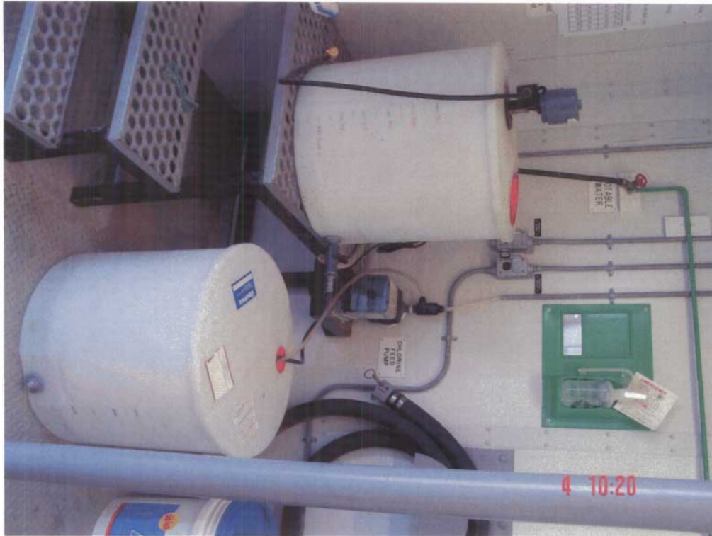
Photo # 3. Chlorination system at Water Intake Facility.
