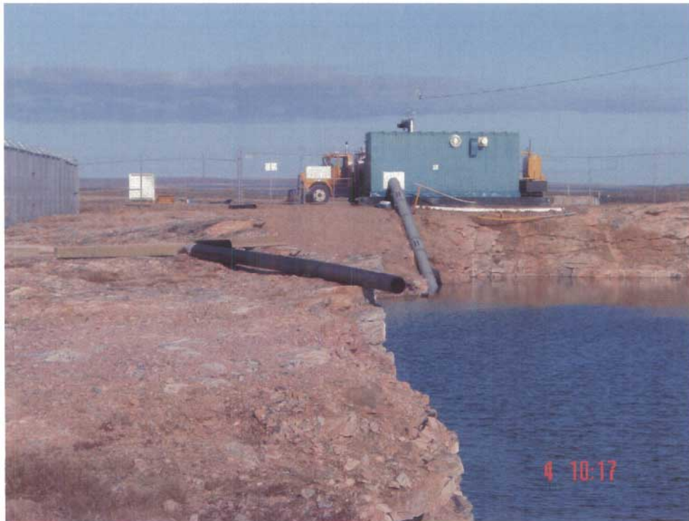
Photo # 2. Water Intake Facility at water reservoir, reservoir fill pipe noted in photo left.
