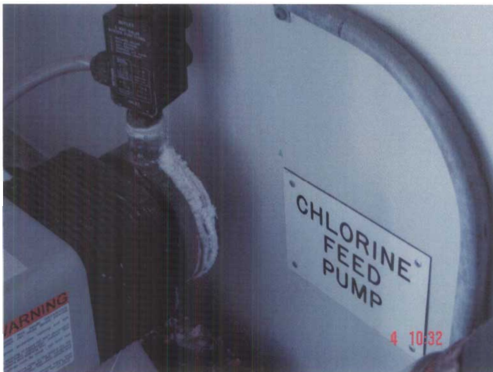
Photo # 4. Chemical feed pump on chlorine concentrate requires maintenance.
