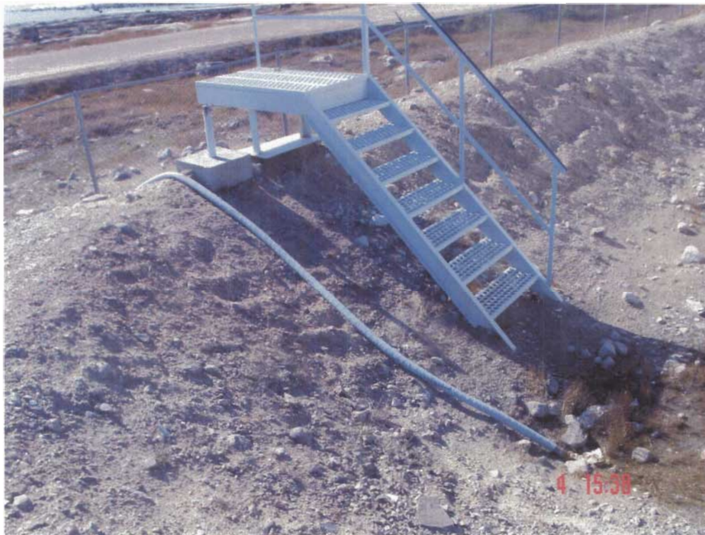
Photo # 16. Drainage hose left unattended in Tank Farm berm.
