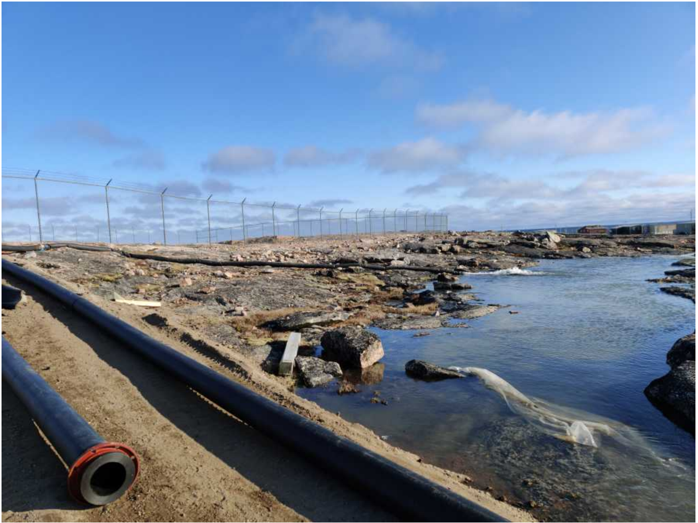
Photo 4: 2:15 pm – Photo taken a station 3+200, facing east. Water first reaches the reservoir-end of pipeline at approximately 1:35 pm. Camlock hose installed on pipe end before reservoir for pipeline flushing was not long enough to extend past the local rocky depression containing the gravel pipe base. Some sloughing of the embankment was noted, and ICL was instructed to repair embankment at a later date.
