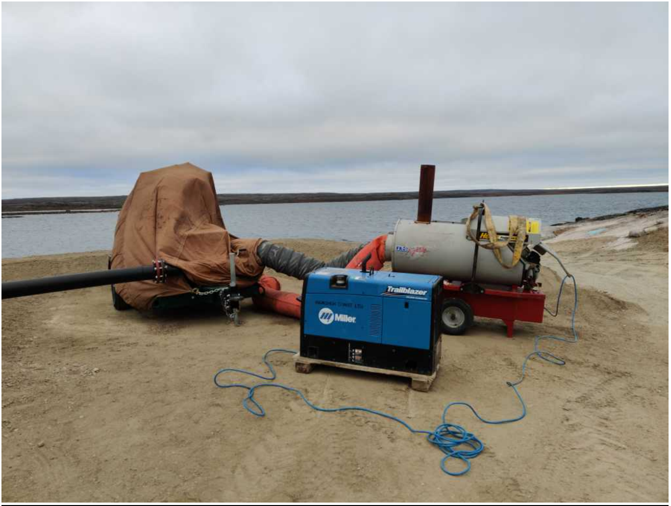
Photo 1: 08:30 am – Heater was installed to ensure pump is ice-free for this afternoon's pump commissioning.
