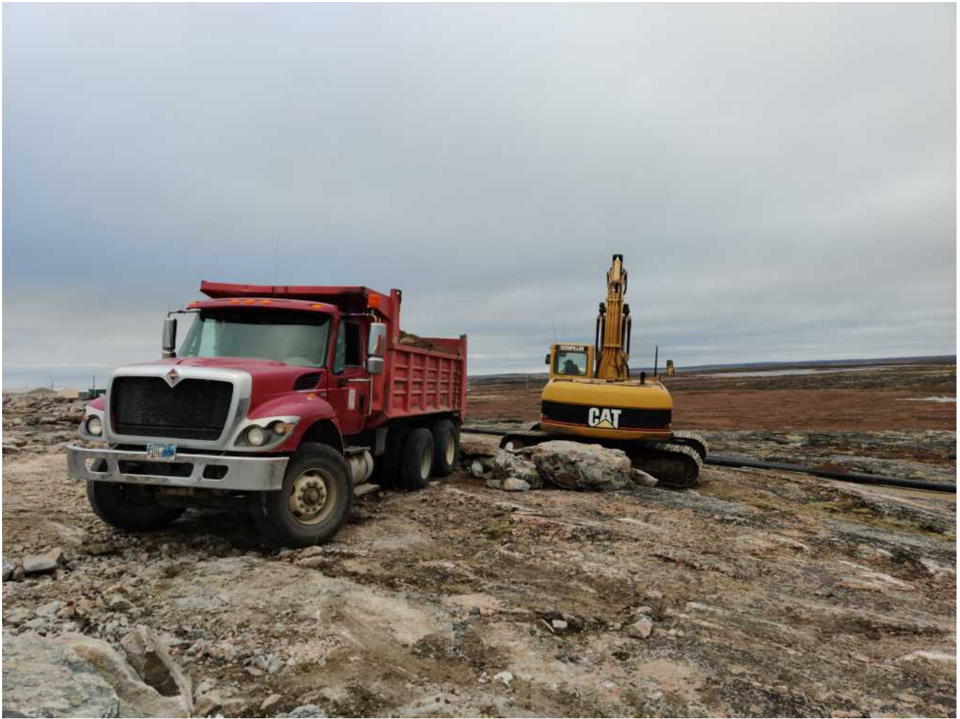
Photo 2: 10:00 am – Photo taken at station 3+000, facing southeast. Berm placement and anchor installation continues from station 3+000. Progress rate slower here due to extra precaution taken to maneuver excavator and dump truck around rocky terrain. By end of day, berm placement and anchor installation reaches station 3+220, with 1 drain valve box installed at station 3+110.
