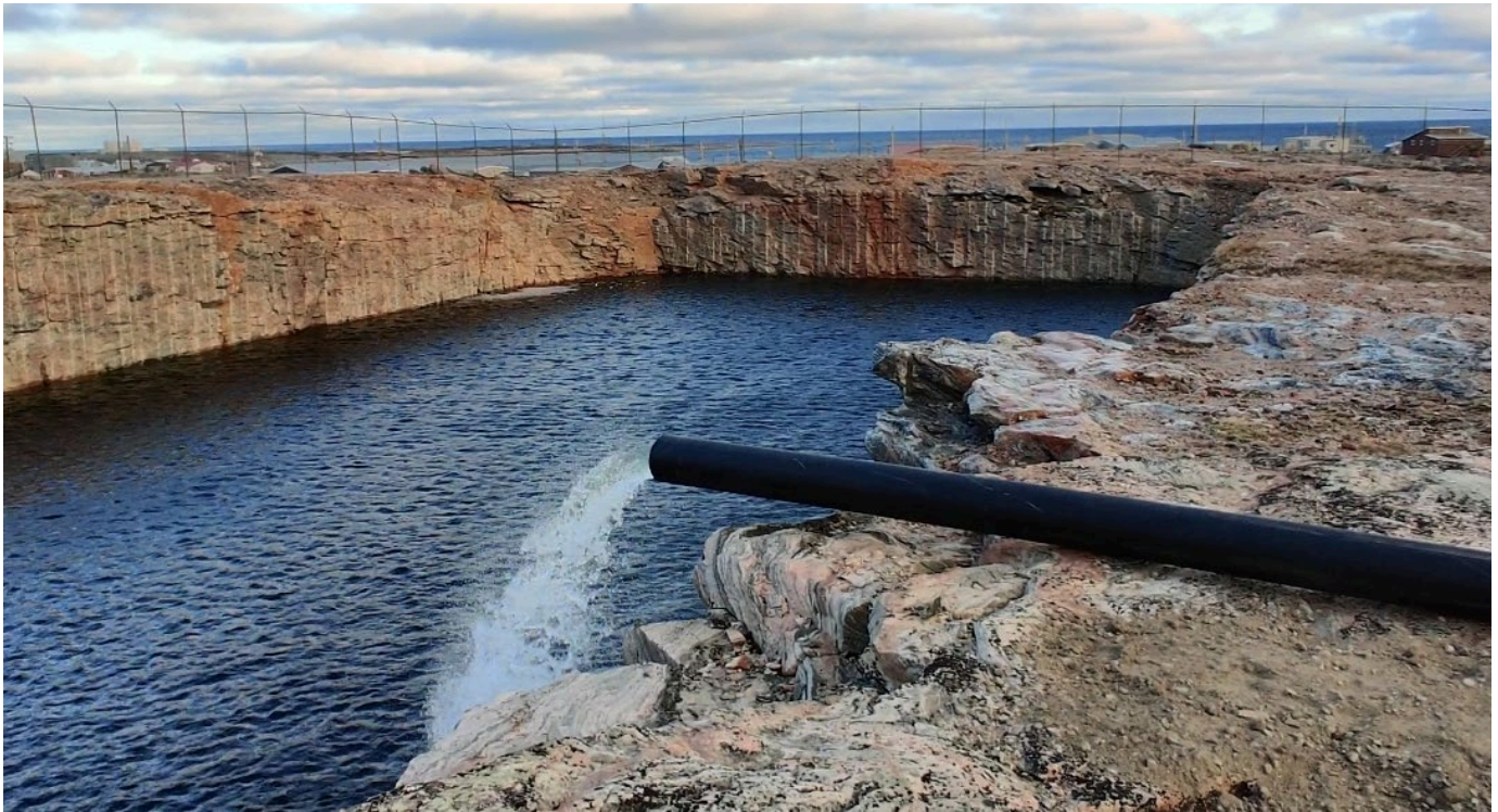
Photo 5: 05:00 pm – Photo taken at reservoir-end pipe outlet. After 1 hour of flushing, crew connected final section of HDPE pipe to the reservoir, and at the request of the Hamlet, pumping proceeded until 7:00 pm to top up the reservoir level. By end of day, 759,859 liters of water were added to the reservoir.
