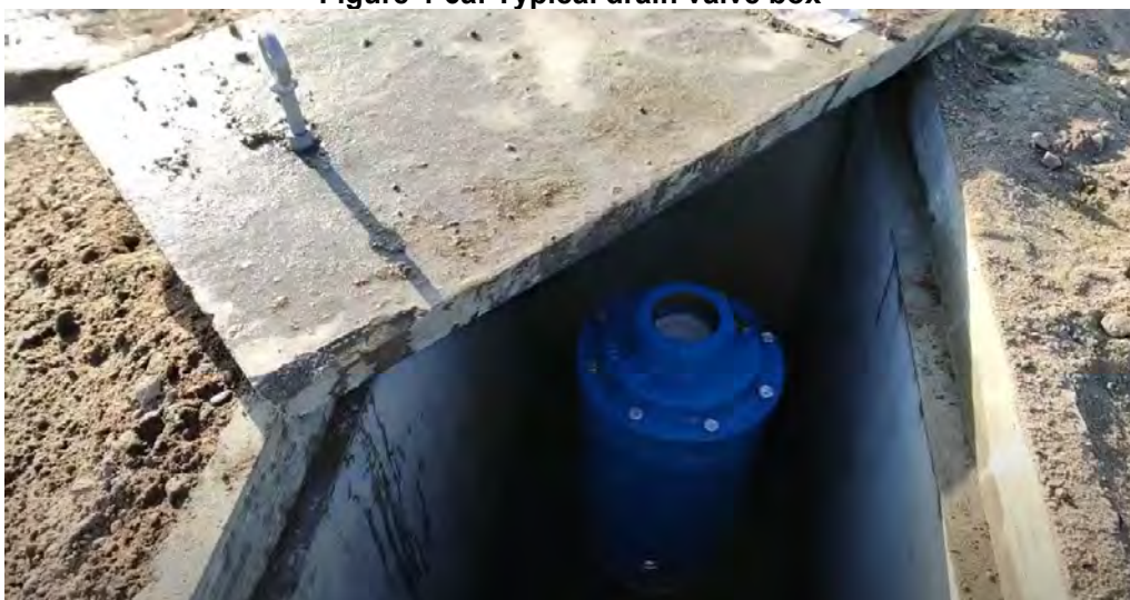
Figure 4-6b: Typical air release valve box
