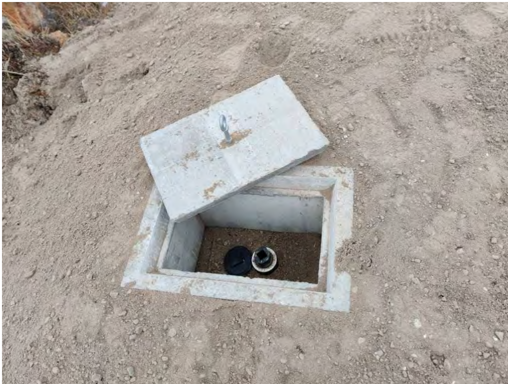
Figure 4-6a: Typical drain valve box
