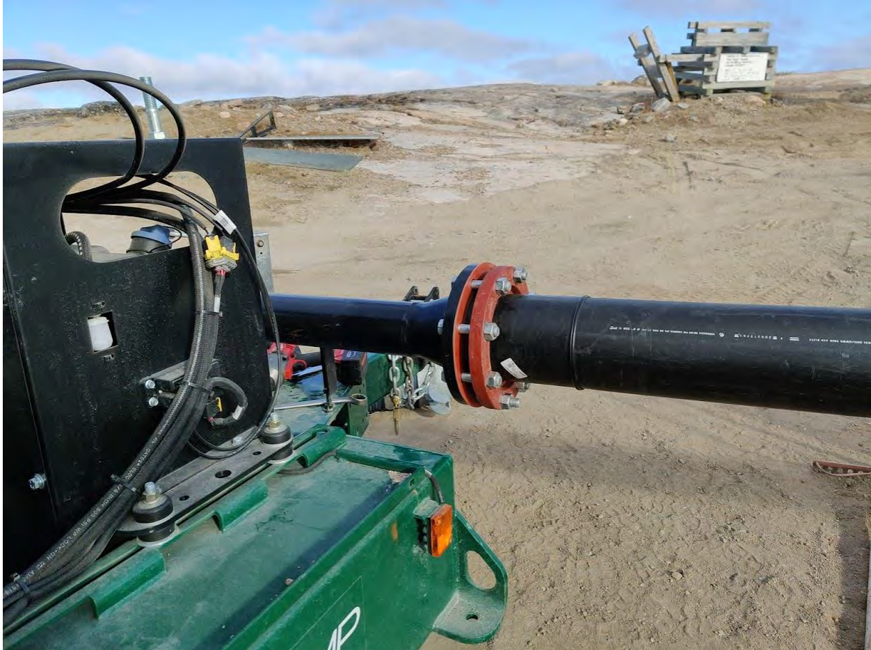
Figure 4-11: Flange connection at pump's tie-in to pipeline. During disassembly, the bolts should be partially loosened to allow trapped water to drain before fully disconnecting the pipe to avoid eroding the pumping pad
