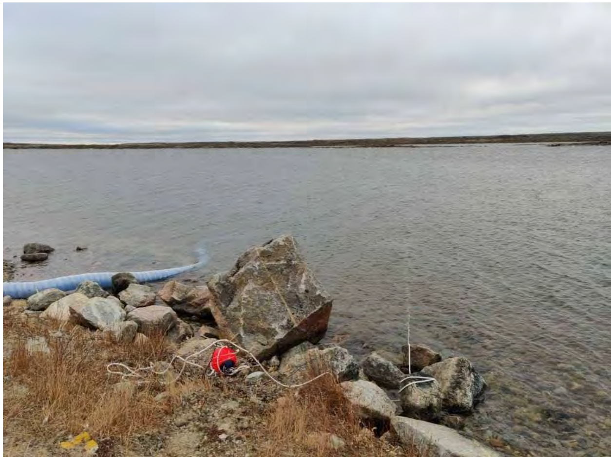
Figure 3-5: Submerged Pump with Attached Rope for Retrieval
