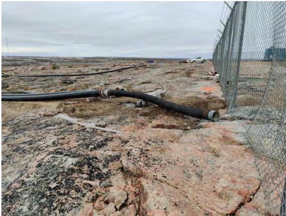
Figure 4-2: Flexible Hose Attached to End of Pipeline During Flushing
