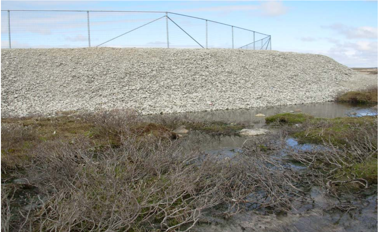
Main effluent seep outside SE corner of lagoon
