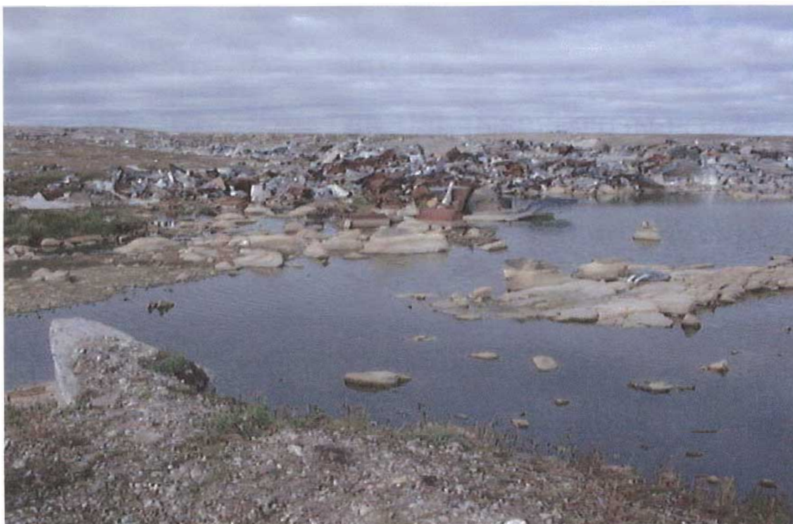
figure 7. Pooled water along the toe of the solid waste disposal facility; 2001/08/24.
