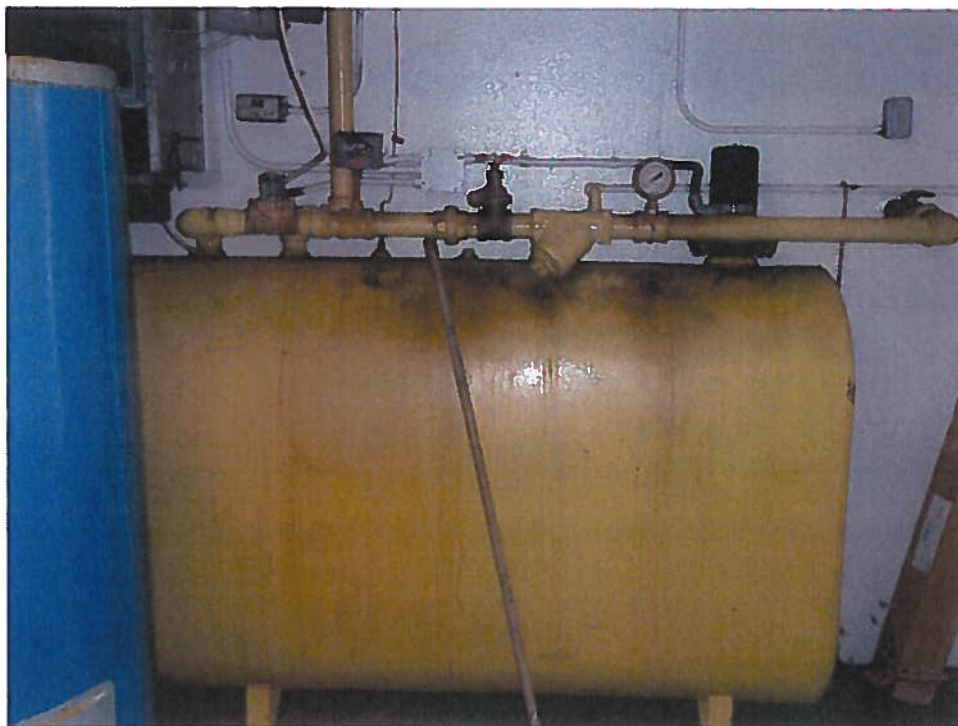
Photo 10: Fuel storage tank inside of pump house
