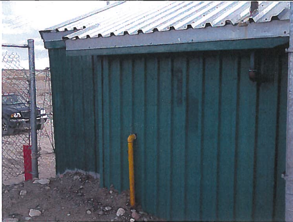
Photo 9: Fuel intake pipe into pumphouse
