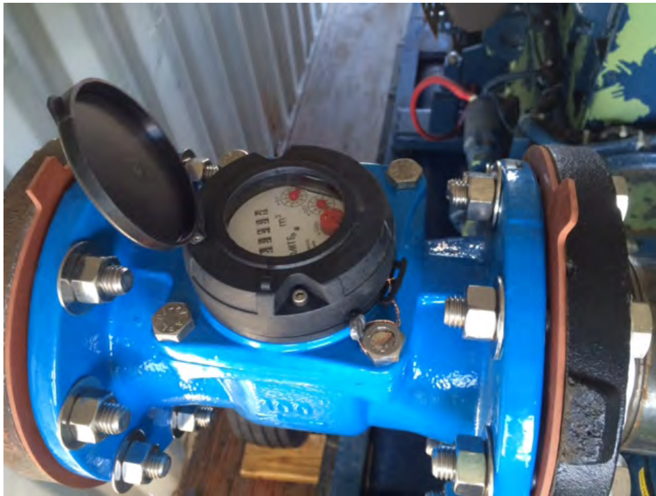
Figure 3: Top View of Flow Meter at Char River
