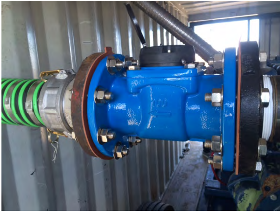
Figure 2: Side View of Flow Meter at Char River
