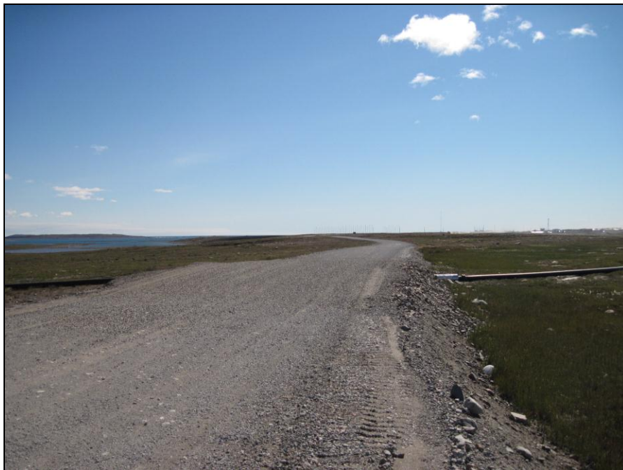
Photo 4: One section of the pipeline crossing under the existing municipal access road.
