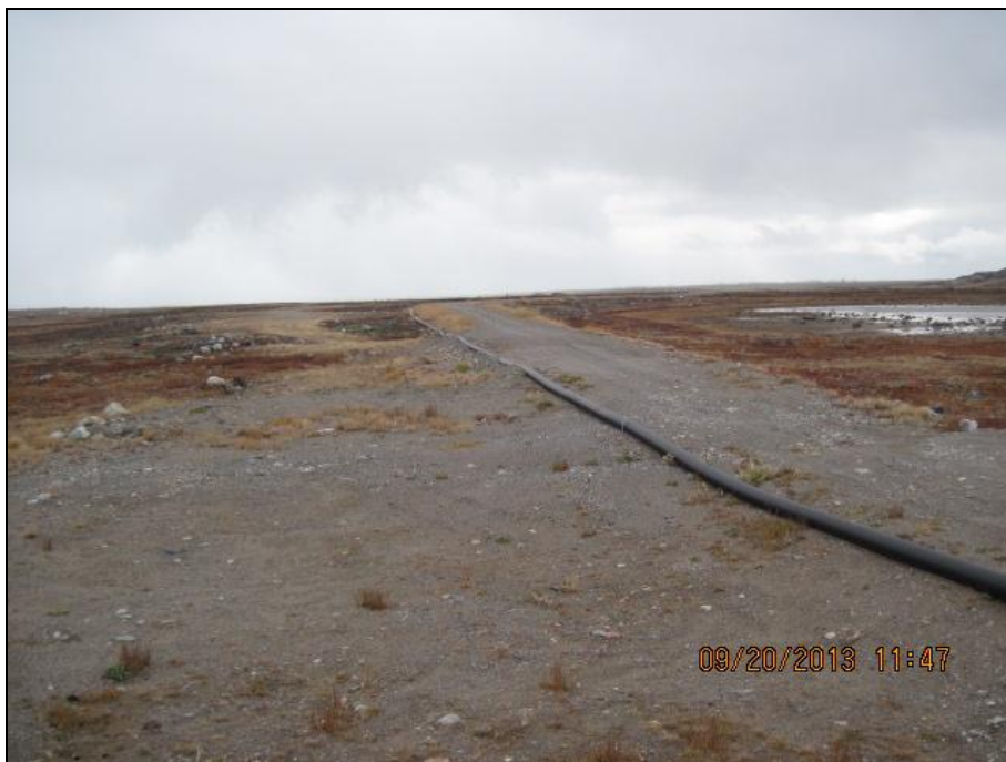
Photo 2: Pipeline traversing land adjacent to access road.
