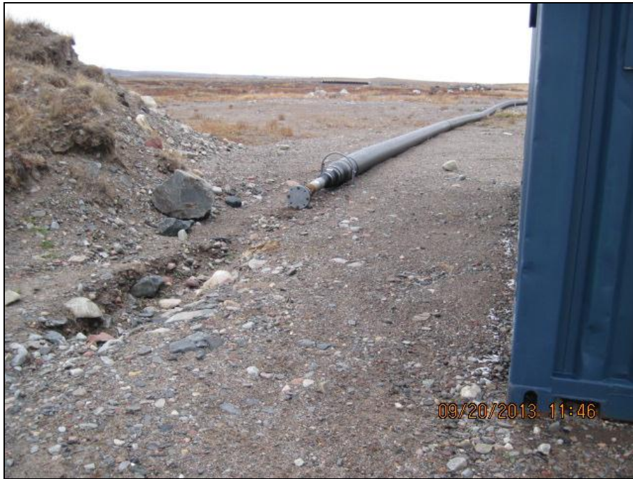
Photo 3: Future location of the pump. Note sea canister in foreground.
