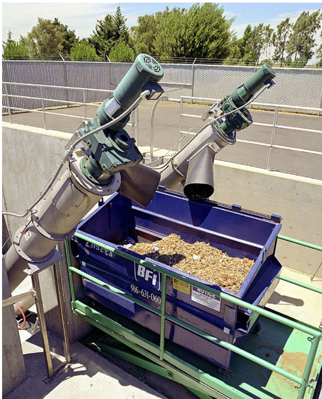
Example of monster auger discharging into BFI roll bin
