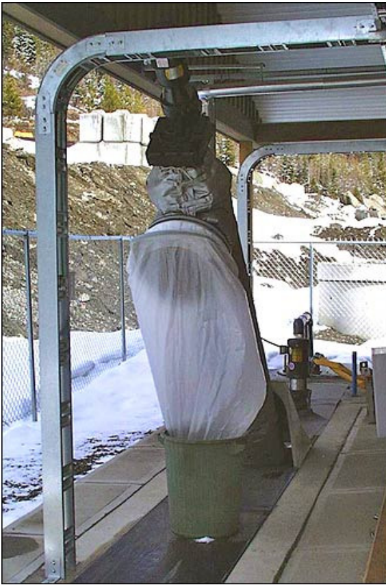
Example of using a bagger collection system.
