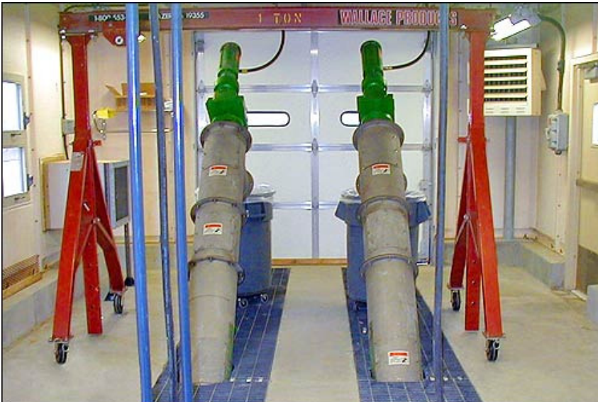
Example of monster auger hoist lifting system
