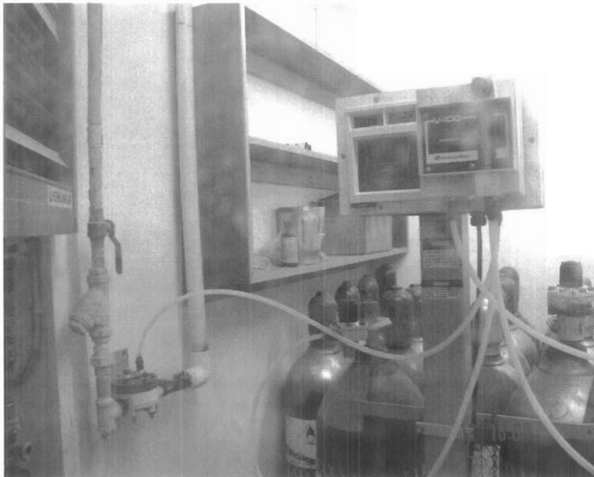
Figure 2. Chlorination system for the Hamlet of Rankin Inlet at Williams Lake treatment plant.
