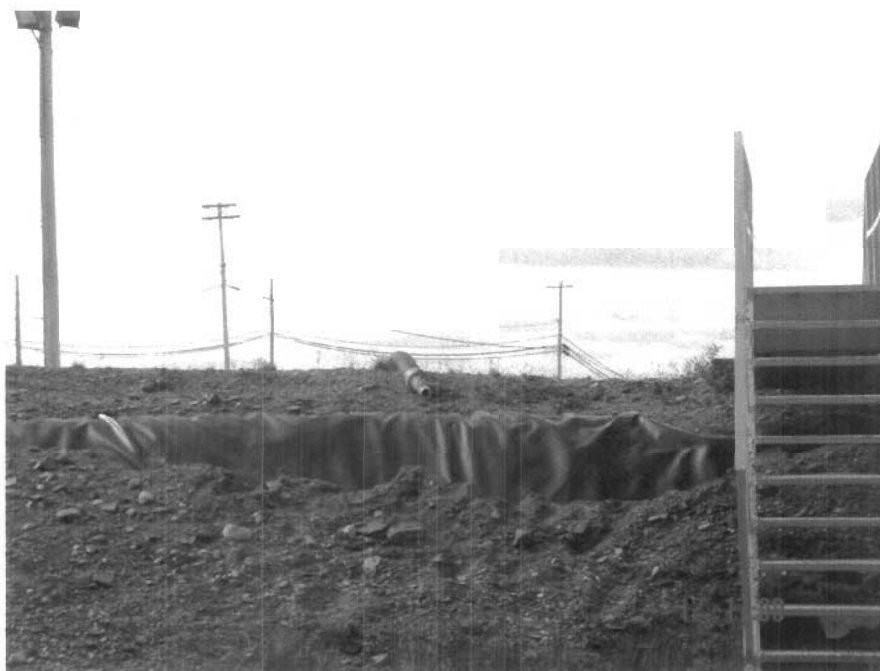
Figure 6. Exposed liner in the berm of the Rankin Inlet Fuel Storage Facility.
