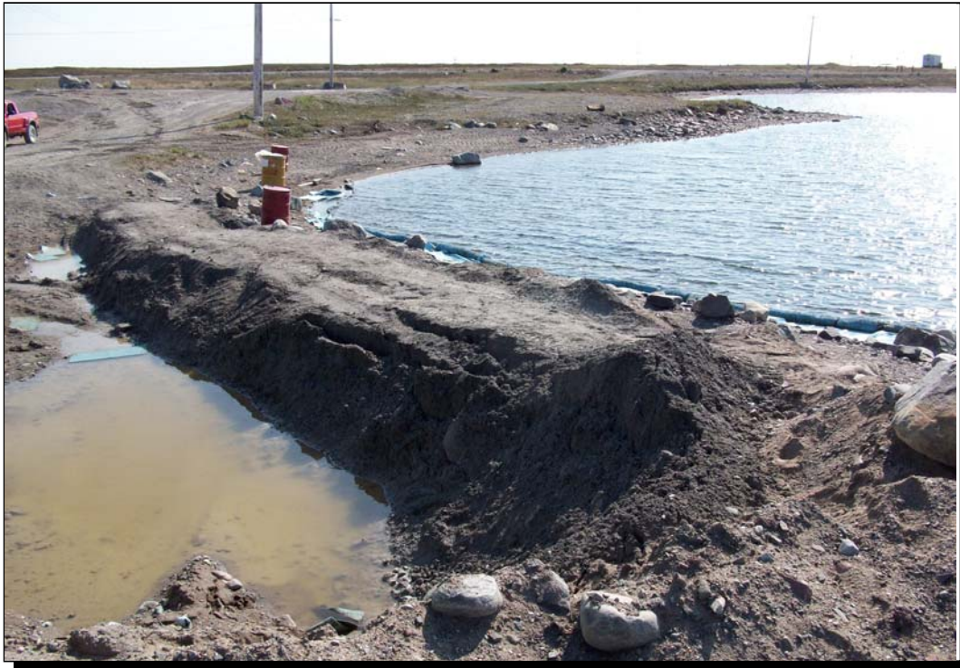
Photo 5 (EBA photo: August 1st, 2008) Clay containment wall
