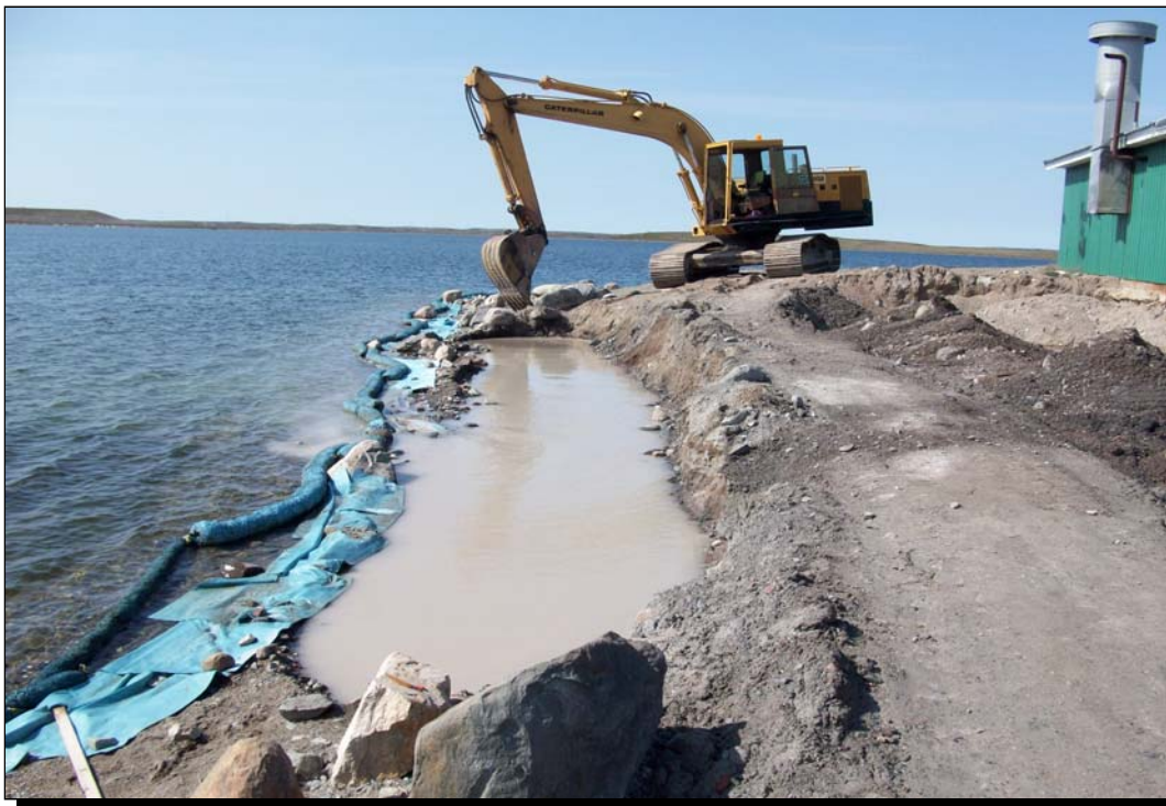
Photo 6 (EBA photo: August 3 rd , 2008) Excavation of beach, south of containment wall
