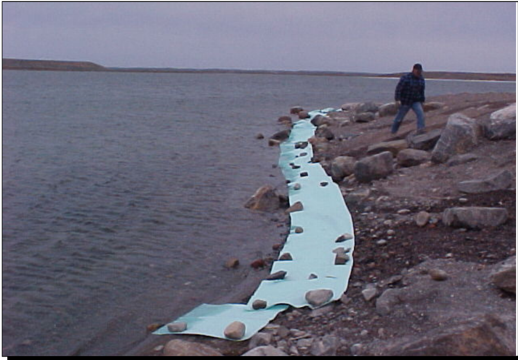
Photo 3 (CGS photo: June 30 th , 2008) Sorbent pads on shoreline
