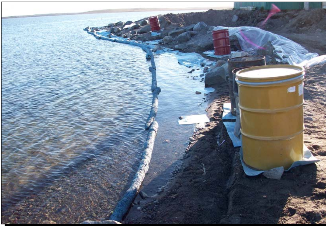
Photo 4 (EBA photo: July 4 th , 2008) Sorbent boom around shoreline
