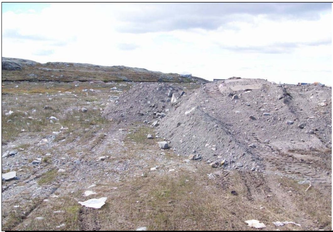
Photo 9 (EBA photo: July 6 th , 2008) Impacted soil stockpile at Rankin Inlet landfill
