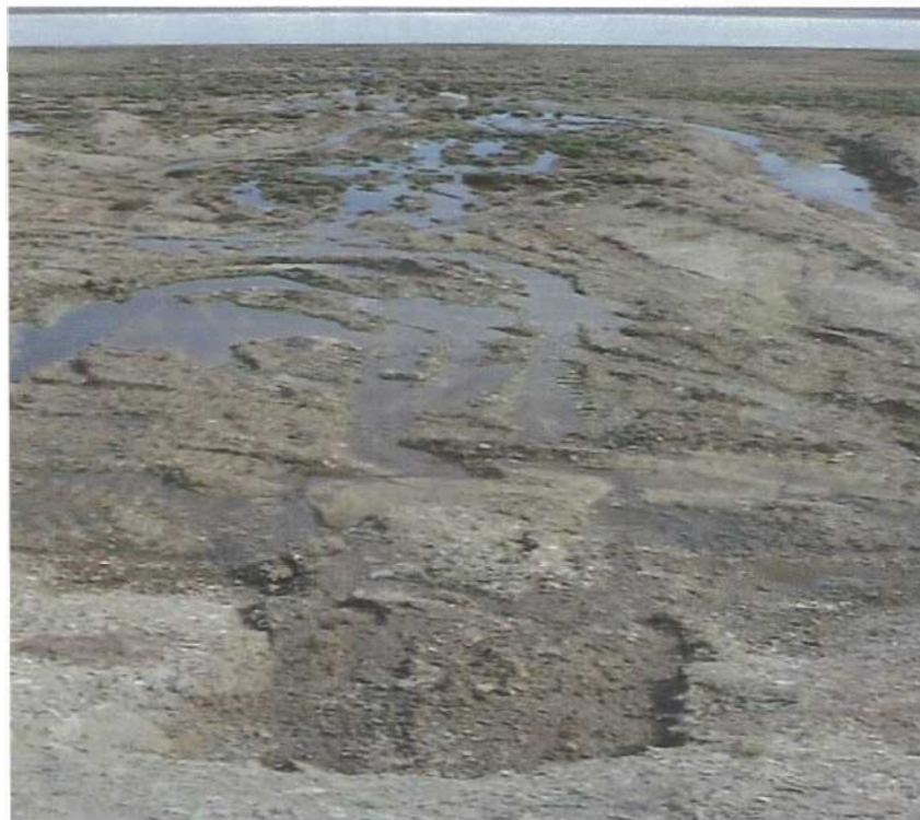
figure 2. Seepage and erosion along the outer face of sewage lagoon cell 2; 2001/07/12.
