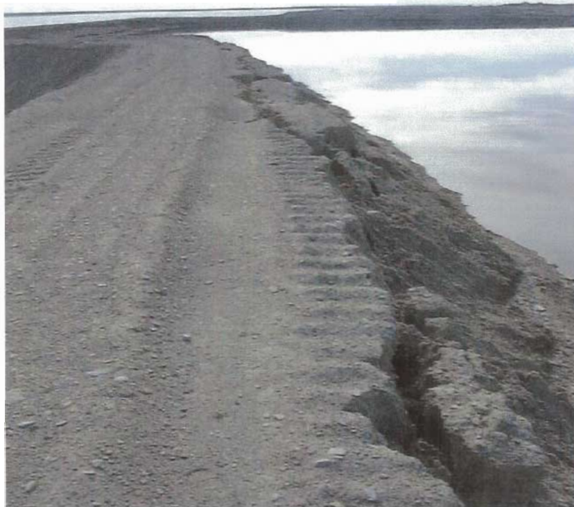
figure 1. Erosion along the inner face of sewage lagoon cell 3; 2001/07/12.
