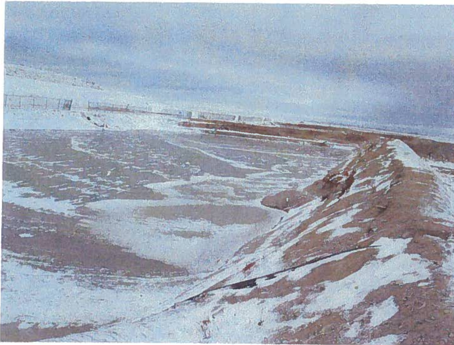
Photograph 3: Lagoon No. 3, looking west towards Lagoon No. 4
