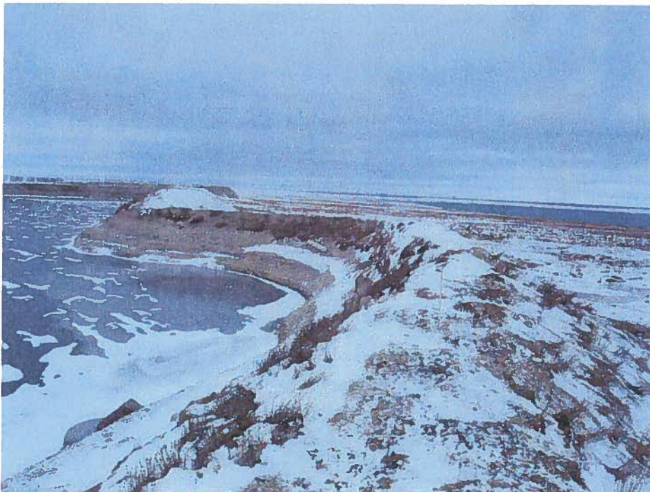
Photograph 2: Lagoon No. 2 berm, overlooking wetland
