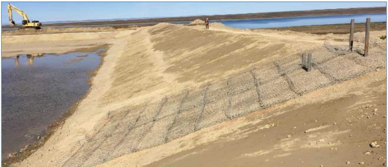
Photo 12: Gabions installed for a discharge chute
