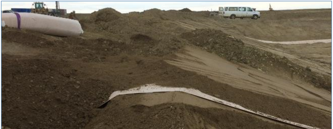
Photo 9: Cell B key to anchor GCL liner
