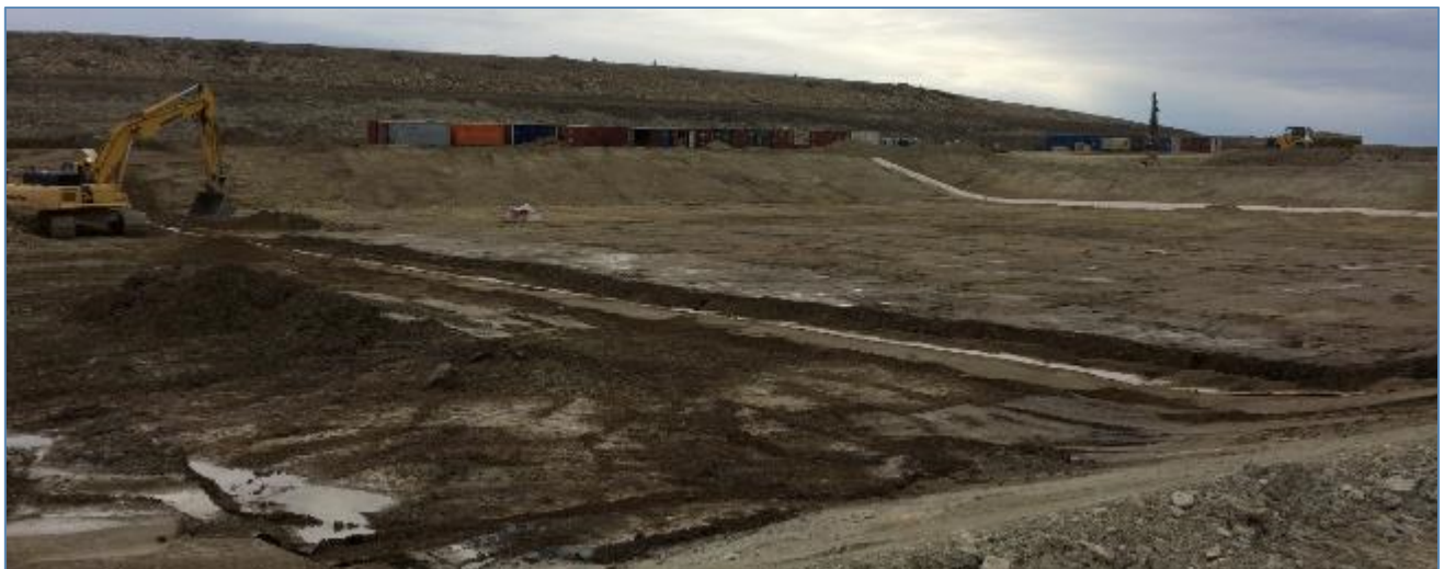
Photo 9: Cell B key to anchor GCL liner
