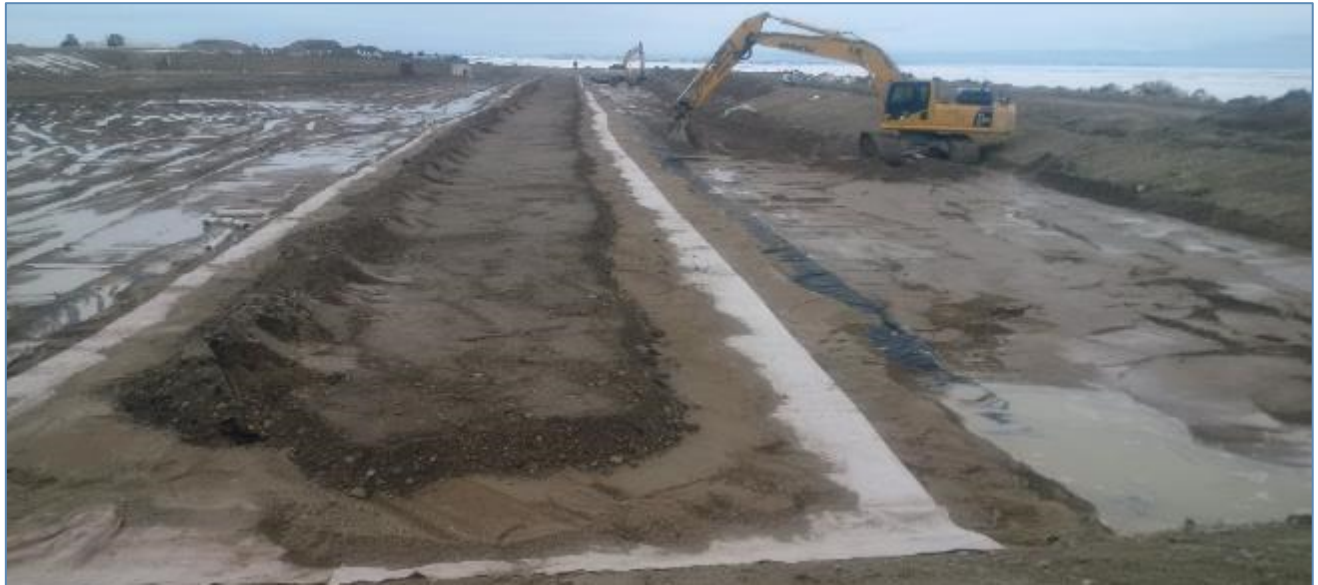
Photo 6: Construction sequence during base construction at Cell A. Visible layers (from the top) include gravel, sand, GCL, sand, woven geotextile and sand.
