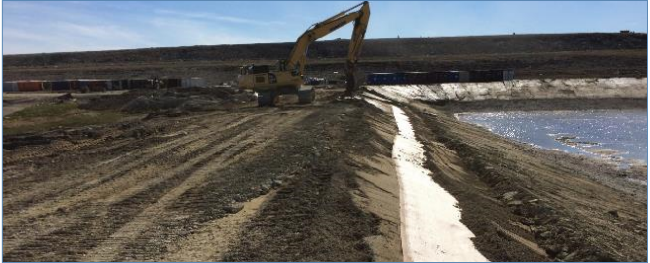
Photo 8: Cell A berm construction
