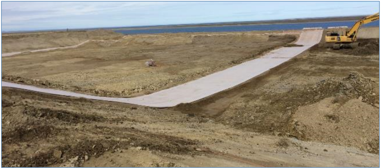
Photo 11: Cell B GCL liner installation
