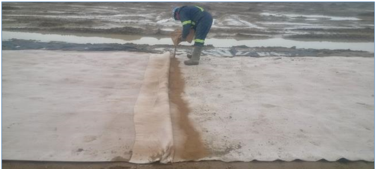
Photo 7: Connecting GLC segments
