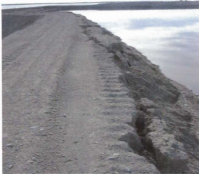
figure 1. Erosion along the inner face of sewage lagoon cell 3; 2001/07/12.
