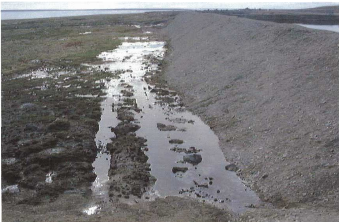
figure 3. Seepage along the outer face of sewage lagoon cell 1; 2001/07/12.
