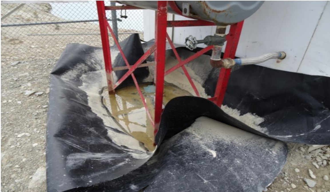
Figure 3 Lack of proper secondary containment at fuel tank adjacent to reservoir
