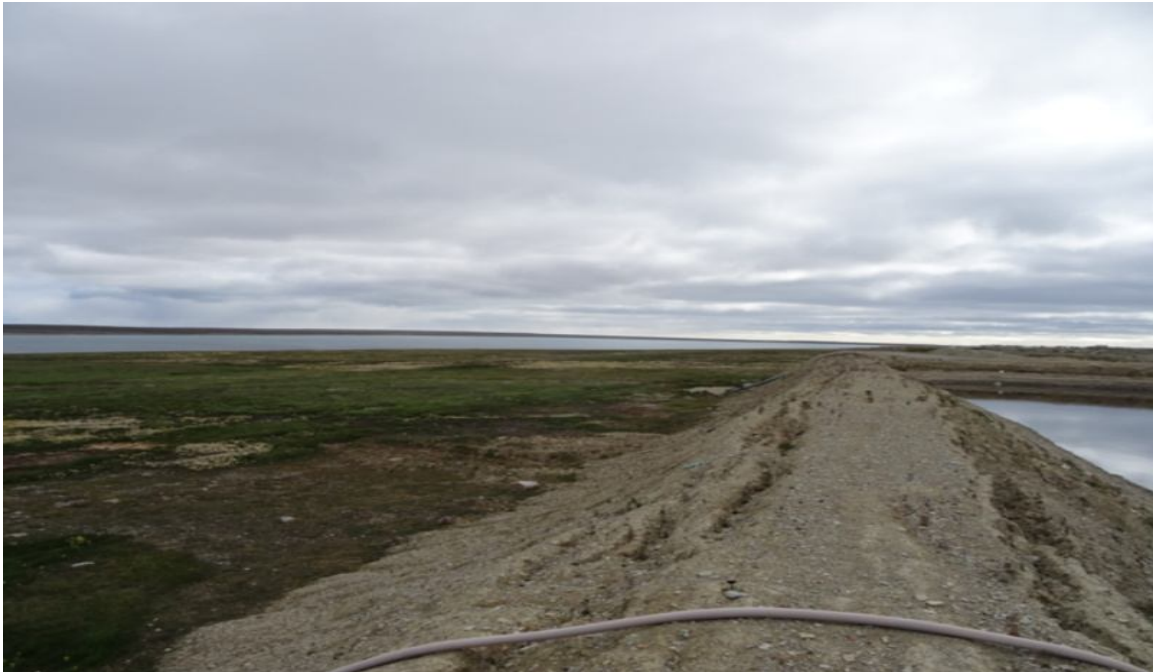
Figure 18 Lagoon wall, erosion and settling, sloughing evident on both faces
