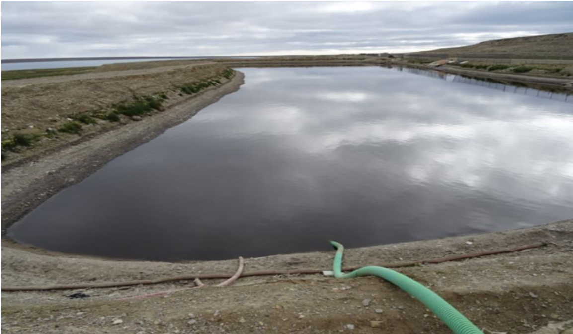
Figure 15 decanting of cell at Lagoon. Lack of a float on suction line allows sludge to be taken up and ejected out of the facility
