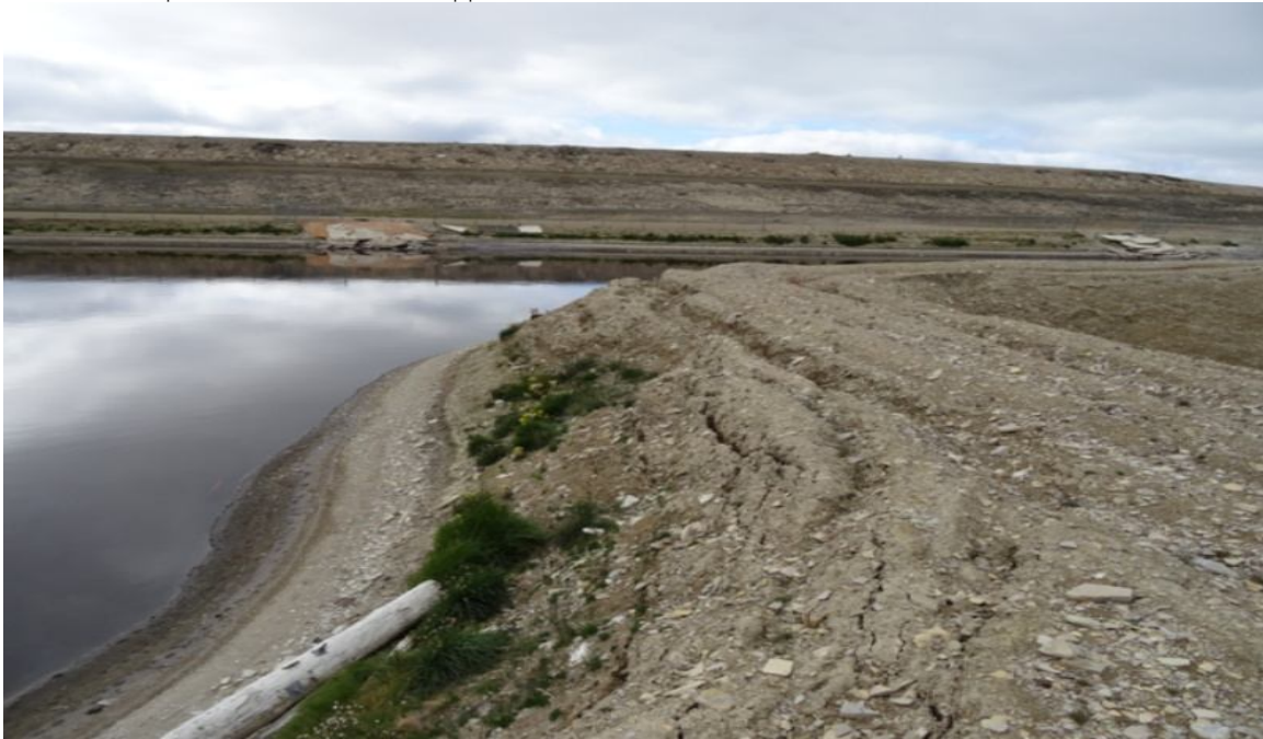
Figure 17 wall of lagoon showing signs of settling and erosion
