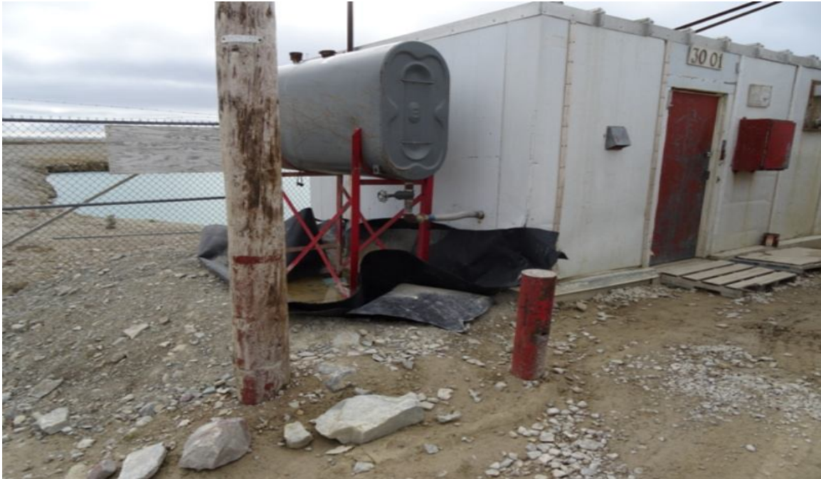
Figure 4 Lack of proper secondary containment
