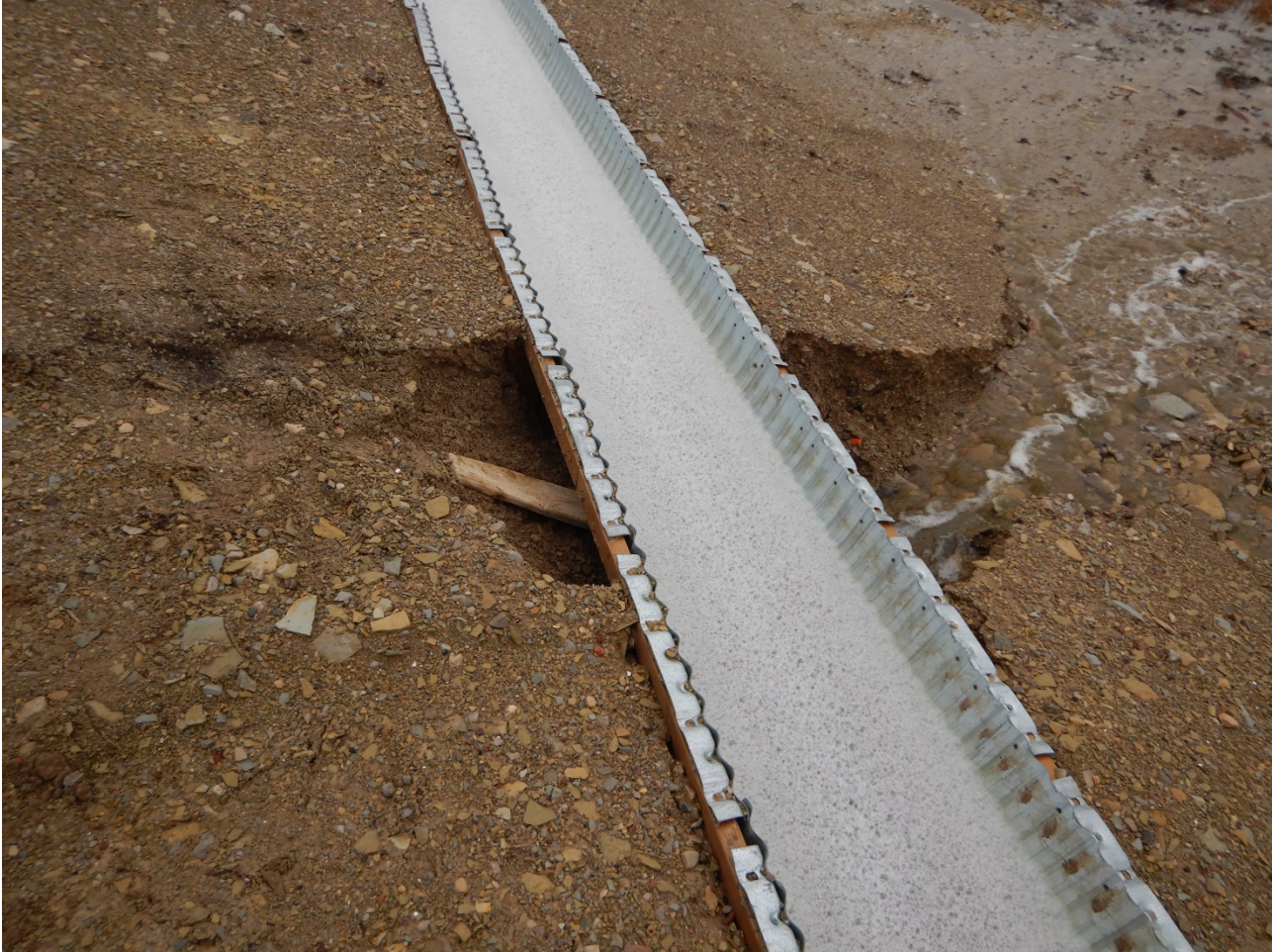
Discharge Location. Half culvert diverting some of the discharge along the intended route. What goes along the half culvert also leaks out and washes out the base of the sewage reservoir.
