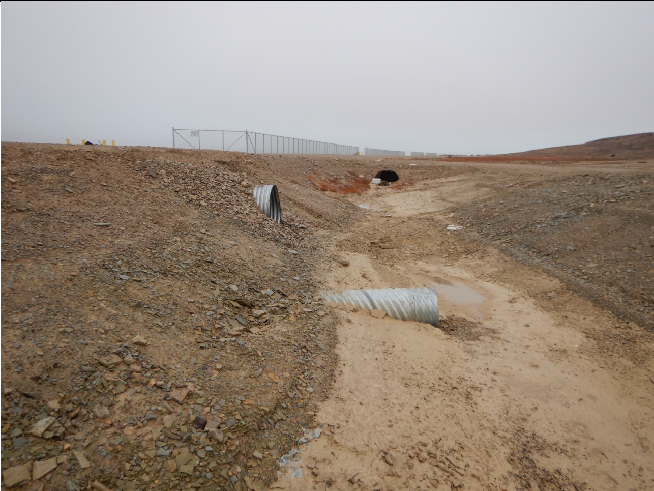
A new Culvert installed to stop the build up of water due to a frozen culvert. Installed spring 2019. The drainage basin appears to be operating as intended.
