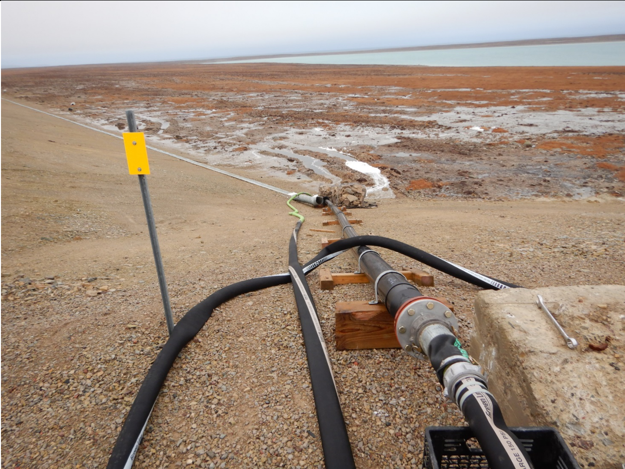
Discharge Location. Half culvert diverting some of the discharge along the intended route. Most of the discharge goes directly to the receiving environment. What goes along the half culvert also leaks out and washes out the base of the sewage reservoir.
