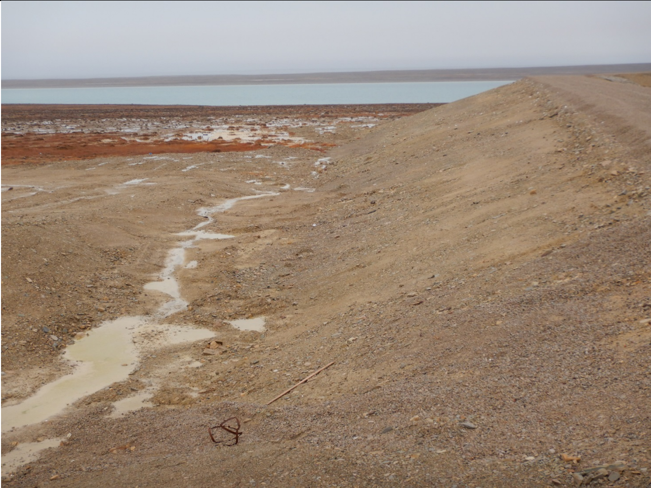
Cell #1 Outer wall of Cell 1 appears to have some minor wheeping.
