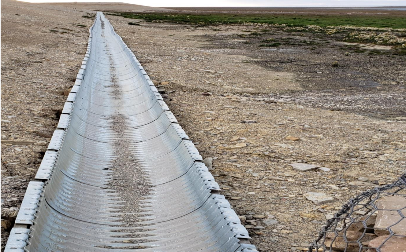
Discharge Location. Half culvert diverting some of the discharge along the intended route. What goes along the half culvert also leaks out and washes out the base of the sewage reservoir.
