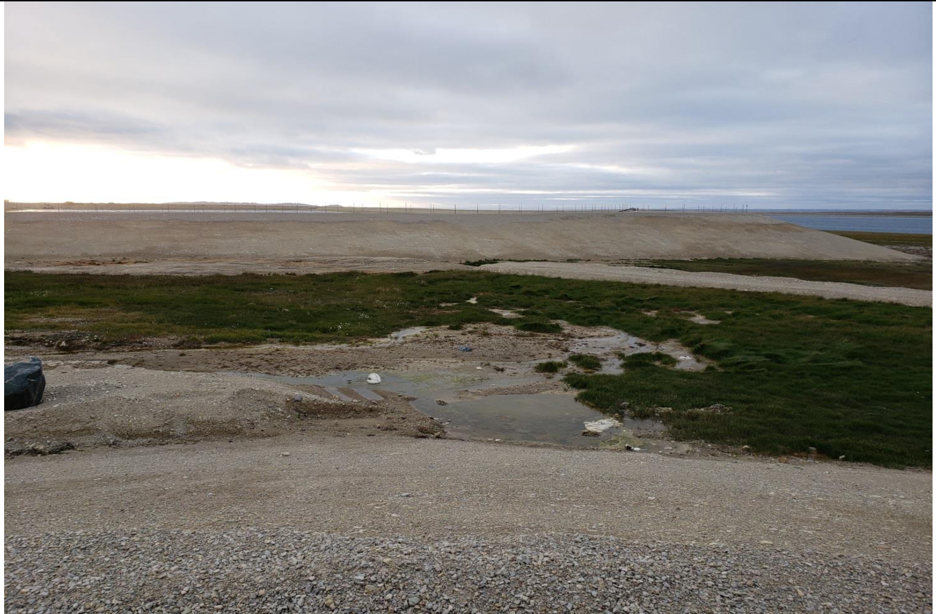
Cell # 2. 2019 signs of slumping may be a leak. Engineer Inspection on walls requested.
