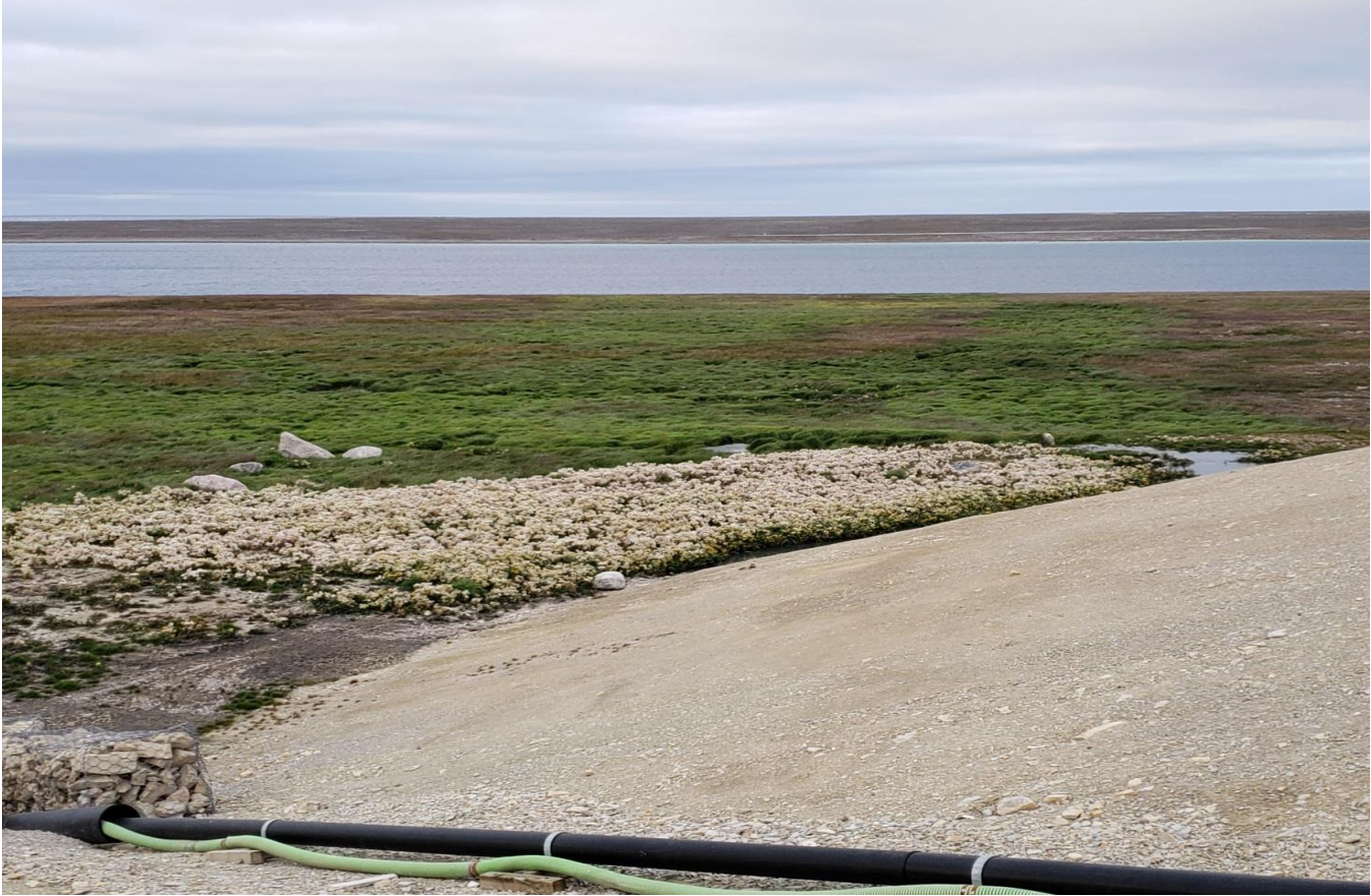
Discharge Location. Half culvert diverting some of the discharge along the intended route. Most of the discharge goes directly to the receiving environment. What goes along the half culvert also leaks out and washes out the base of the sewage reservoir. Dicharge Location for Cell #2
